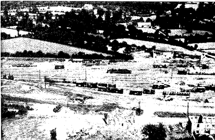
Bomb damage to Folligny Marshalling Yards, France, 8 August 1944.
