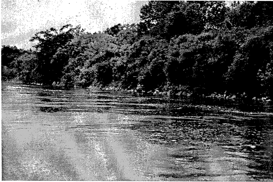
Figure 6. A combination of riprap in the toe section and woody vegetation on the upper banks often affords the best combination of stabilization and environmental benefits
