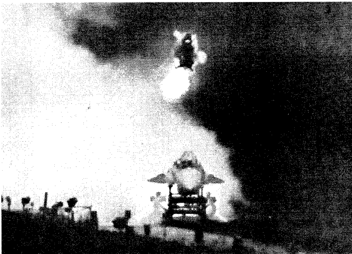
Figure 19. Rocket Sled with Su-27
