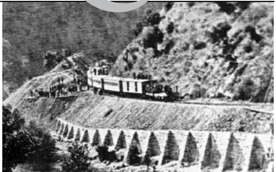
Niles Canyon Railroad. On October 2, 1866 an inspection party visited the Western Pacific Railroad's tracks in today's Niles Canyon. The Western Pacific's inability to finish this railroad through the canyon and on to Sacramento led to a decision to run the transcontinental railroad into Oakland, giving the East Bay ferries a near monopoly on getting passengers into San Francisco.
