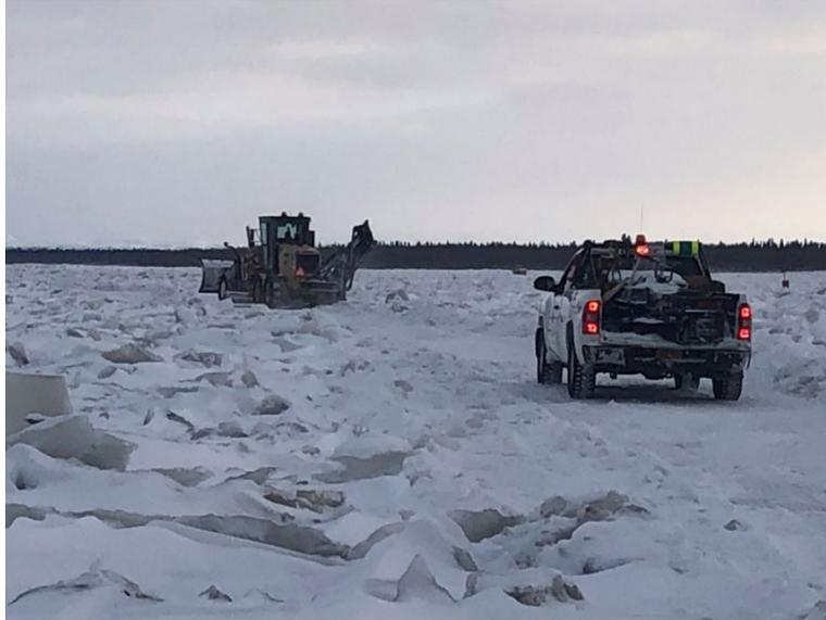
Figure 6.5 Constructing an ice road in rough ice (Image courtesy of Mark Leary, Bethel, AK)
