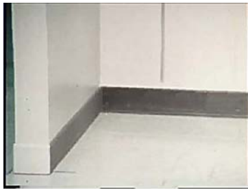
Corner of a room
