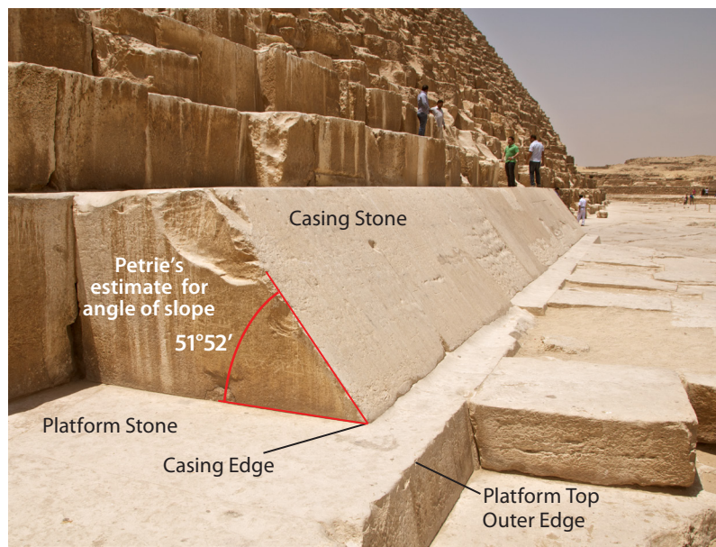
Casing and Platform Stones. Near the corner of the north side the angled casing stones sit upon platform stones. The lower, outer edge of the casing and the top, outer edge of the platform provide the best places to measure the Pyramid's lines. Petrie estimated the angle of the casing slope to be 51^{\circ} 52 \text{ minutes} \pm 2 \text{ minutes} . Photo by Mark Lehner.
