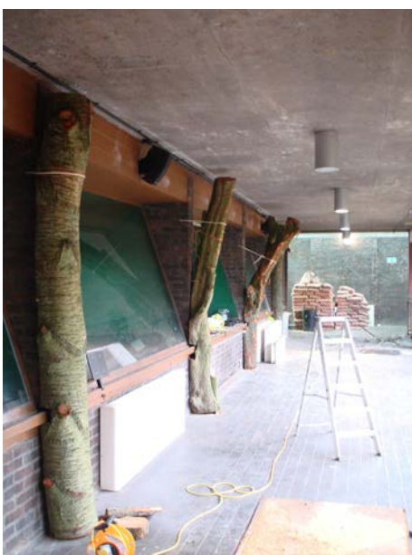
Below: work on the public areas
