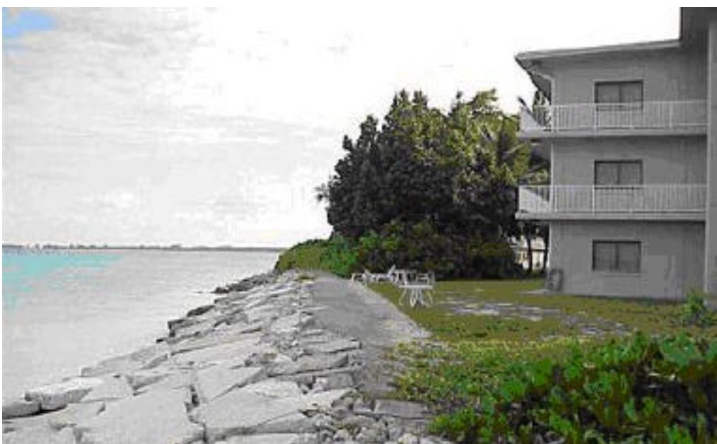
Figure 7.3. Use of concrete for shore protection in northwest Diego Garcia, needed in place of removed vegetation. Taken from (172).
