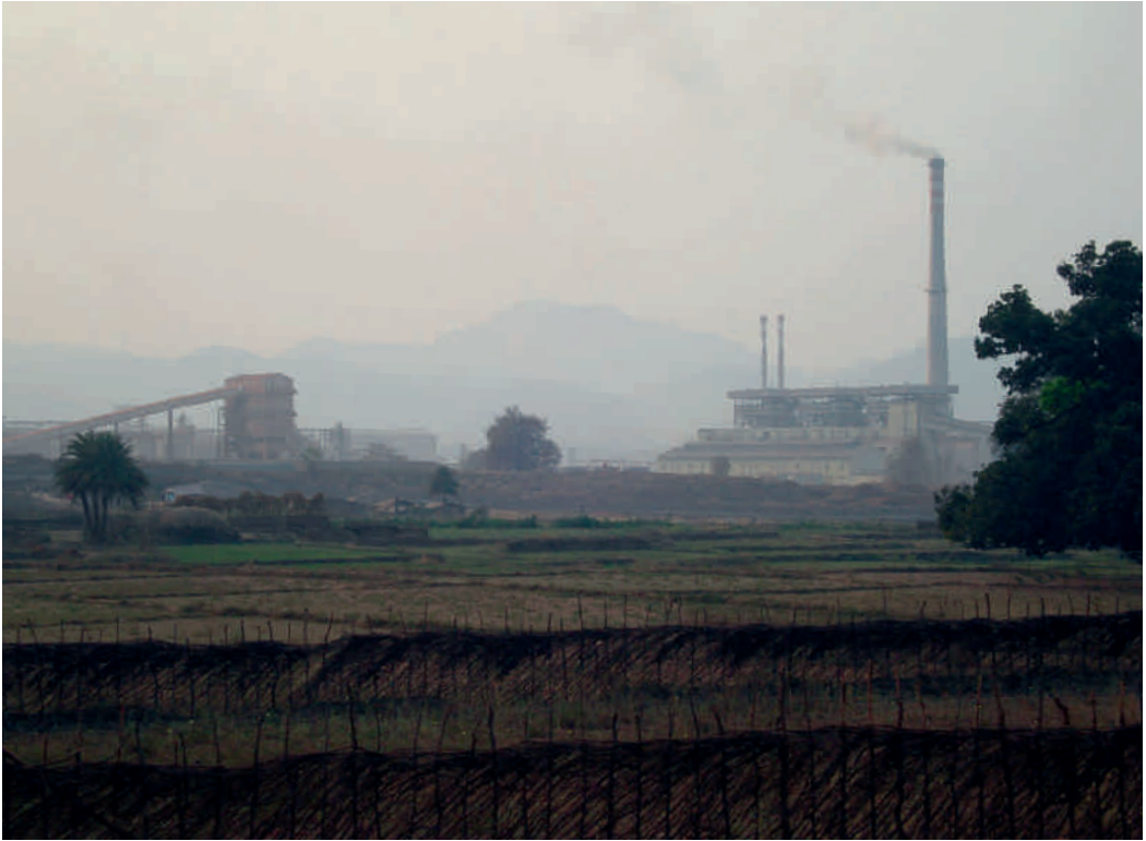
The refinery in Lanjigarh has already displaced three villages completely and is affecting more than 26 villages with its pollution.
