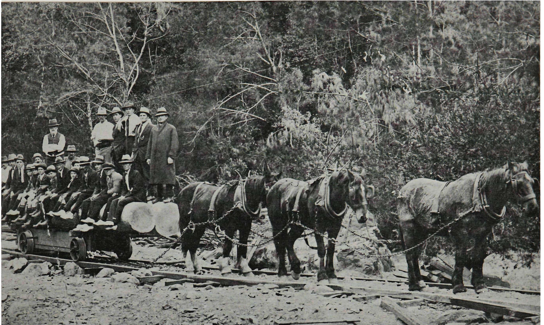
Opening Day, Cressbrook Creek.
