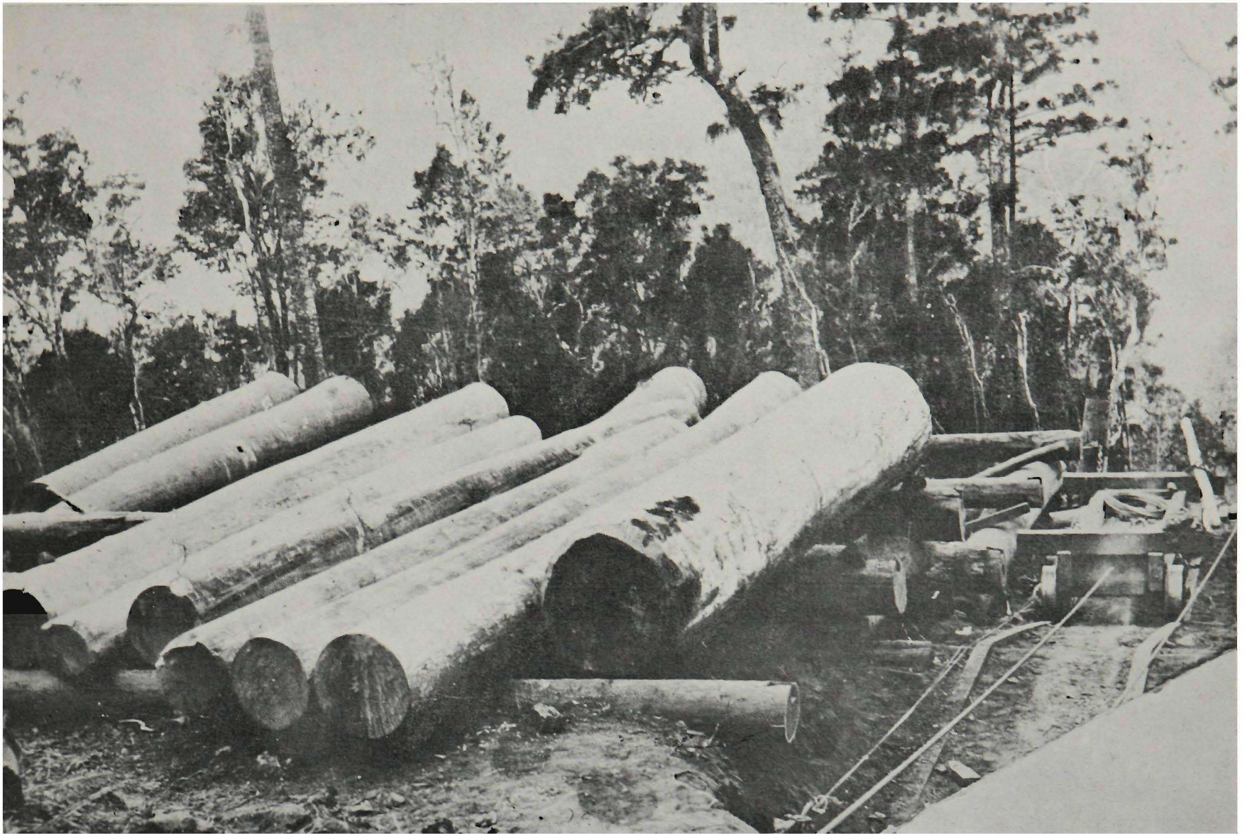
Log Ramp, Cressbrook Incline.
