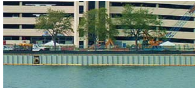
Composite Seawall, Tampa, FL
