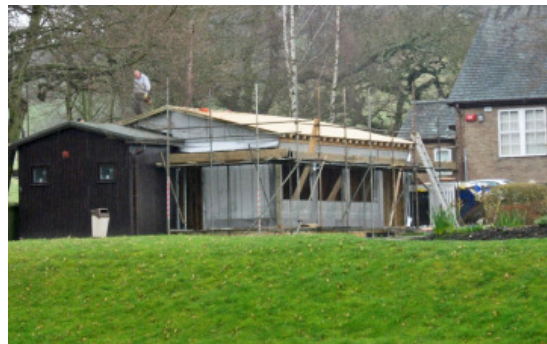
Working on the roof of the pavilion
