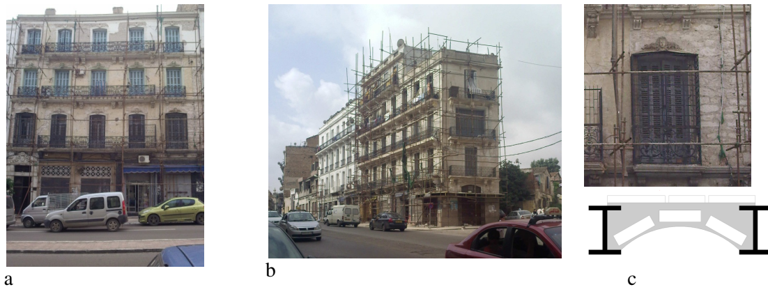
Figure 2. Typical M3.3 buildings (a&b) and details of slab(c)
