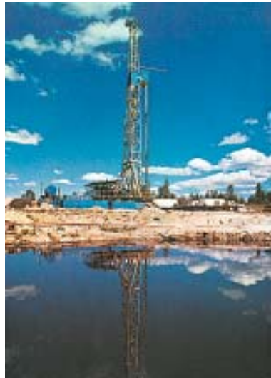
Figure 1. Fenton Hill site. Photo: Courtesy of Los Alamos National Laboratory.
