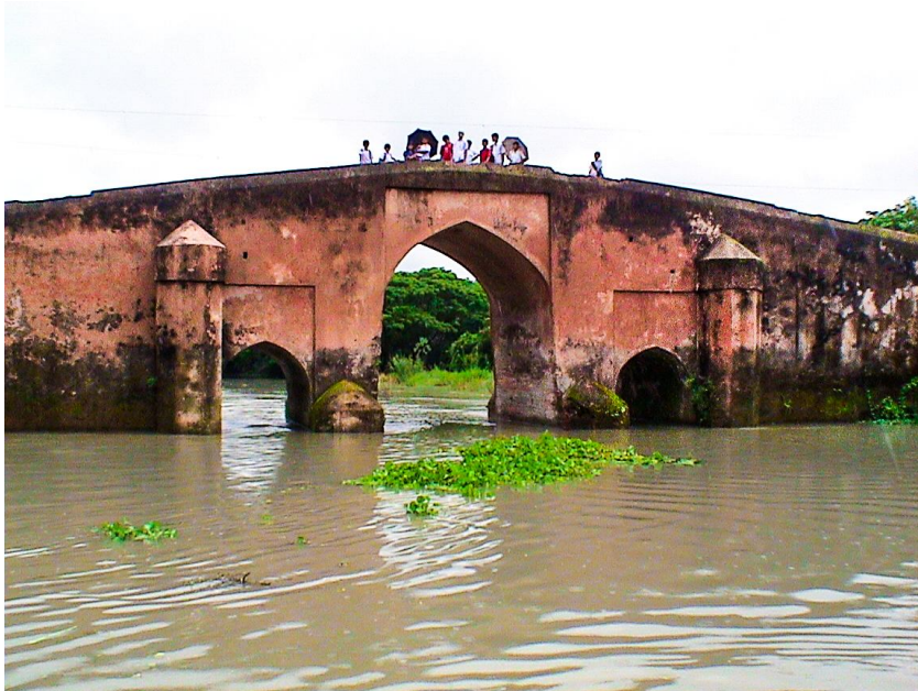
Figure 1. Bridge over the Mir Kadim Canal, Munshigonj
