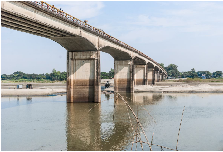
Figure 9. Tora Bridge, one of the first PC girder bridges in Bangladesh
