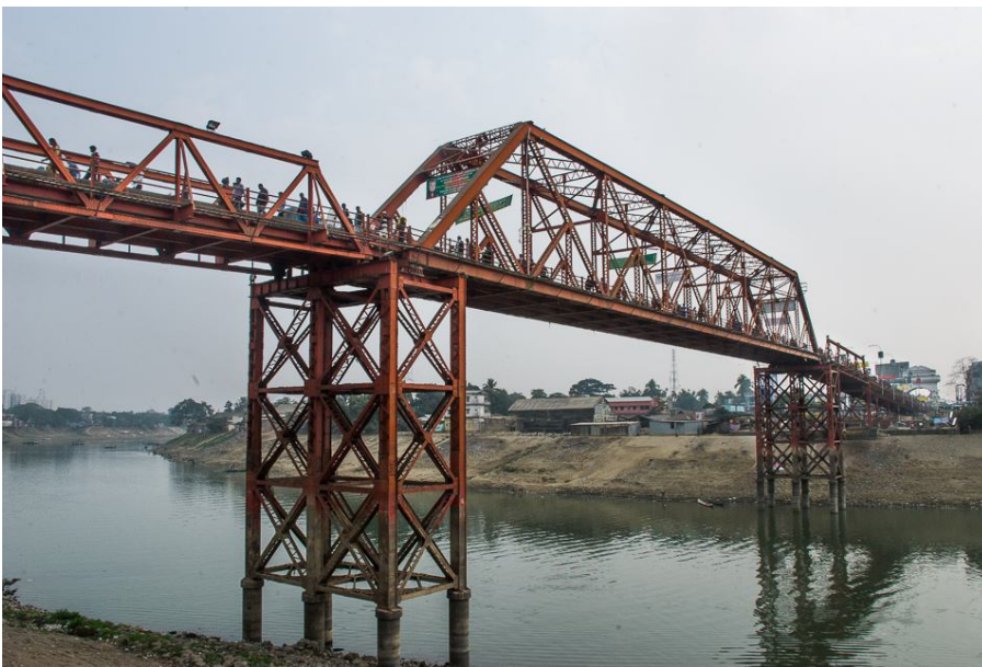
Figure 15. Keane Bridge, Sylhet
