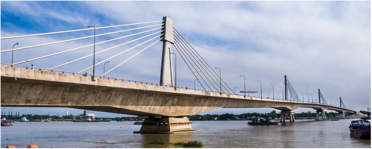
Figure 14. Third Karnaphuly Bridge
