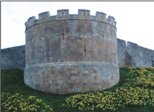
Robin Hood's Tower
