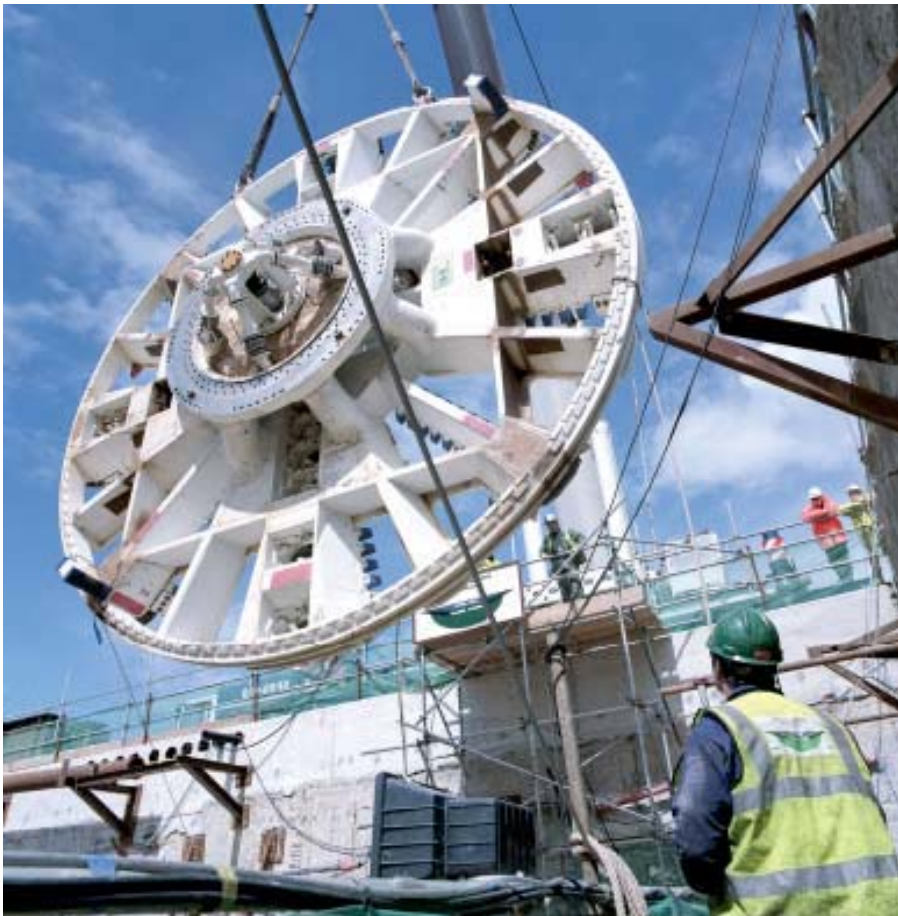
Figure 11: CTRL involved significant tunneling work
