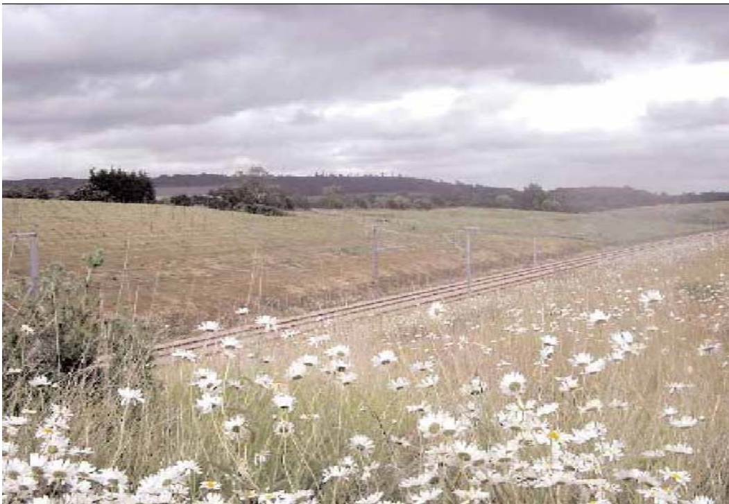
Figure 163: Section 1 of CTRL is finally complete
