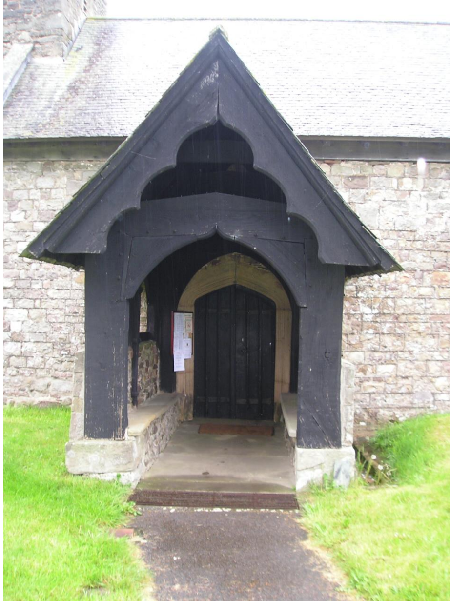
25. St Peter's Church Bryngwyn: woodwork of porch
