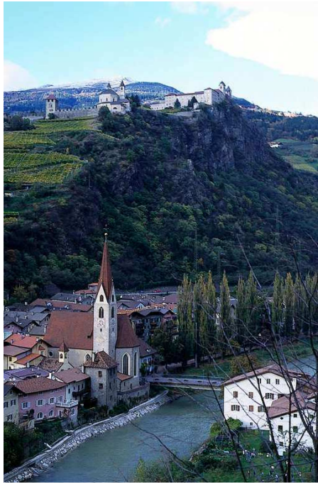
The bridge at Klausen. The Messner’s house is the tall grey one by the river, this side of the church.
