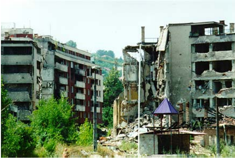
City Damage (Sarajevo)
