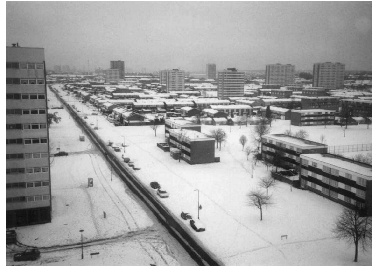
View of Farnborough Road from Vulcan House c1979.
