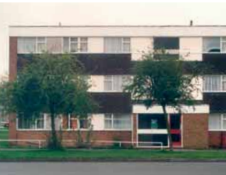
Typical 1960s built walk-up block of flats.
