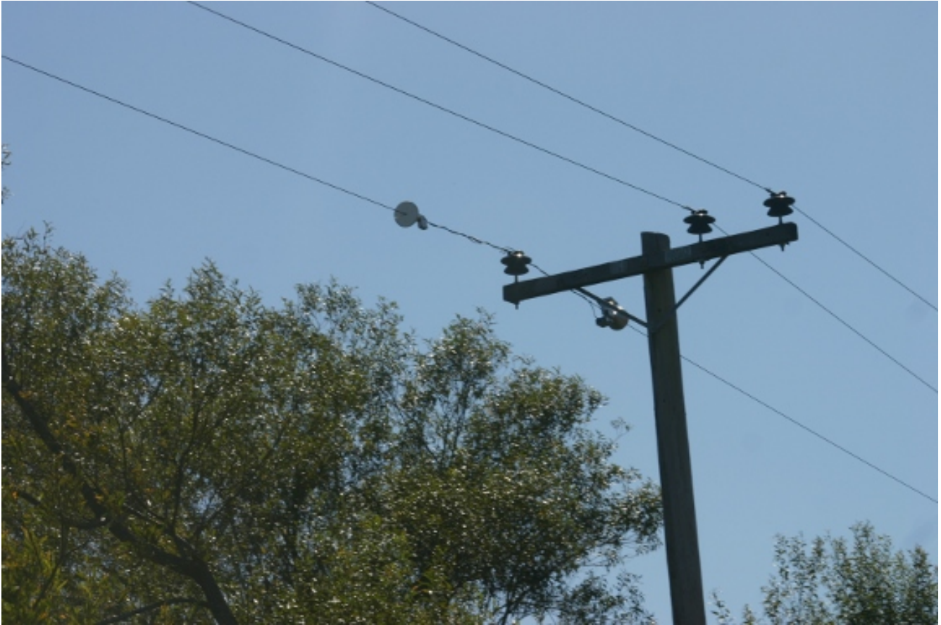
Illustration 12: Photograph of one amplifying node in a prototype system installed on an existing medium voltage power line
