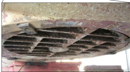
Intakes and Outlets
