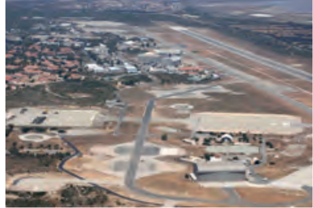
Aerial view of Sovereign Base Areas Credit: Crown Copyright (Ministry of Defence)
