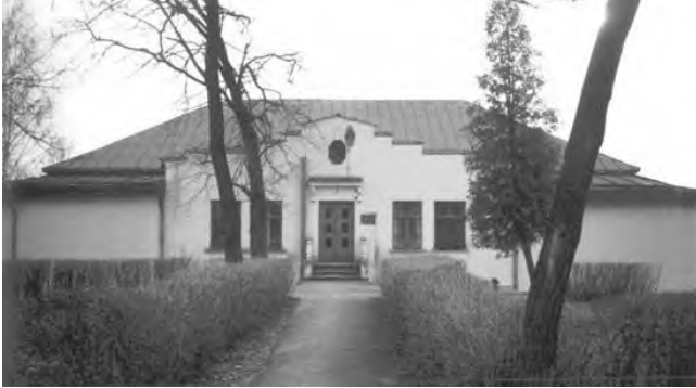
Transmitter building of the "Object Nr. 603" in Kaunas, Lithuania.
