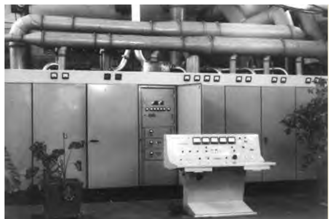
500 kW MW transmitter "Vikhr" was a reserve unit for jamming at Sitkūnai radio station in Lithuania.
