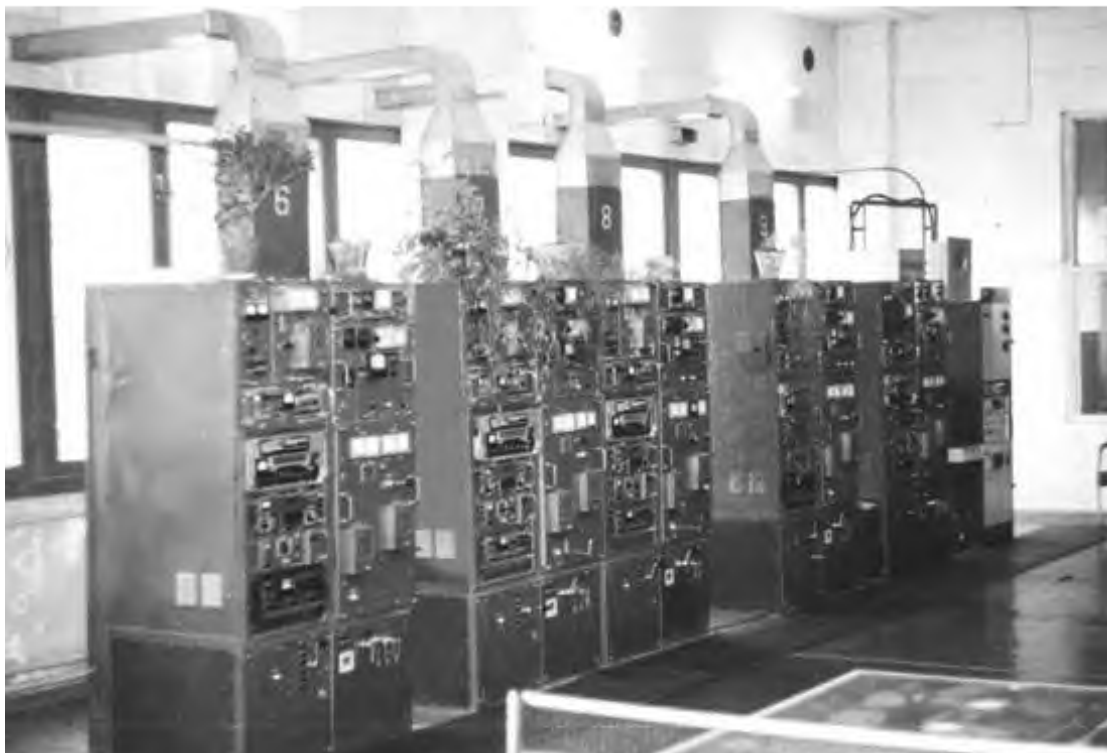
2.5/5 kW SW communications radio transmitters "Viaz-M2" at the local radio jammer near Panevėžys in Lithuania.
