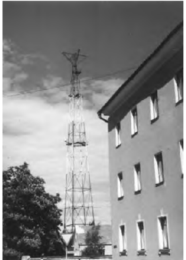
Tower of the local radio jamming station in Tallinn, Estonia.
