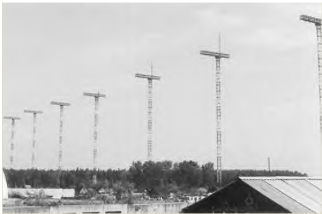
Balashikha local radio jamming station (15x20 kW) near Moscow.
