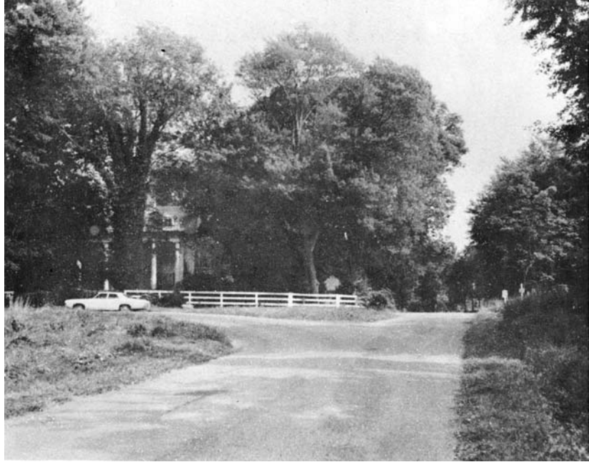
Figure 13. Intersection with the Old Fredericksburg Road Near Shadwell.
