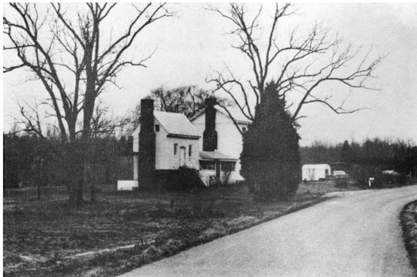
Figure 8. The Tavern at Hadensville.
