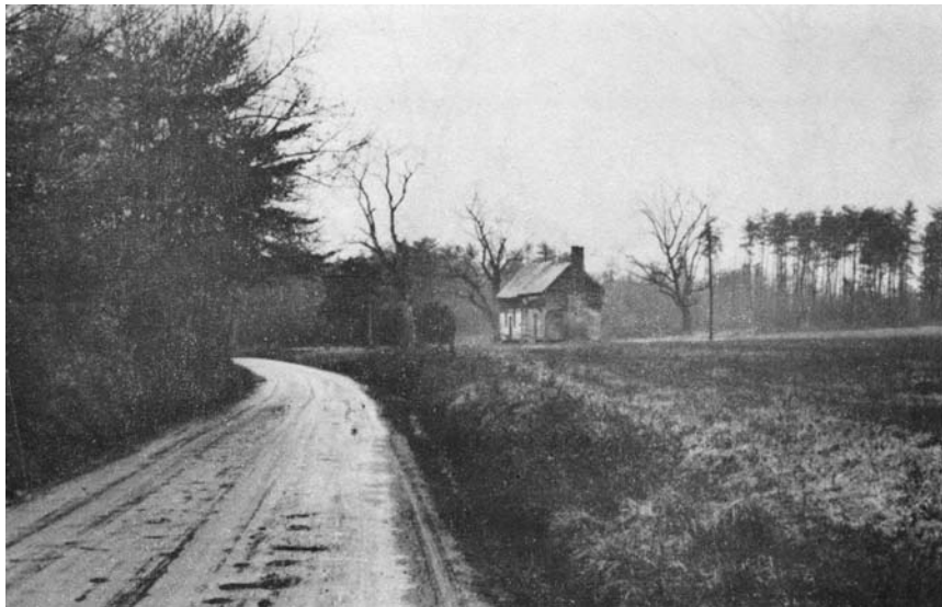
Figure 6. A Portion of Typical Roadbed.
