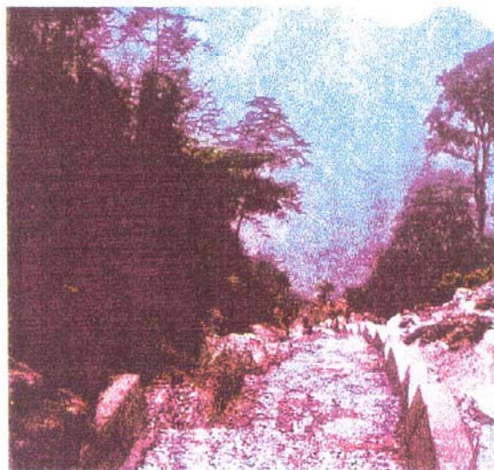
Jhora Training Works of Rafong Khola
