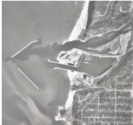
Figure 2. Goderich study area, shown in a 1965 air photo following 1964 record low levels.
