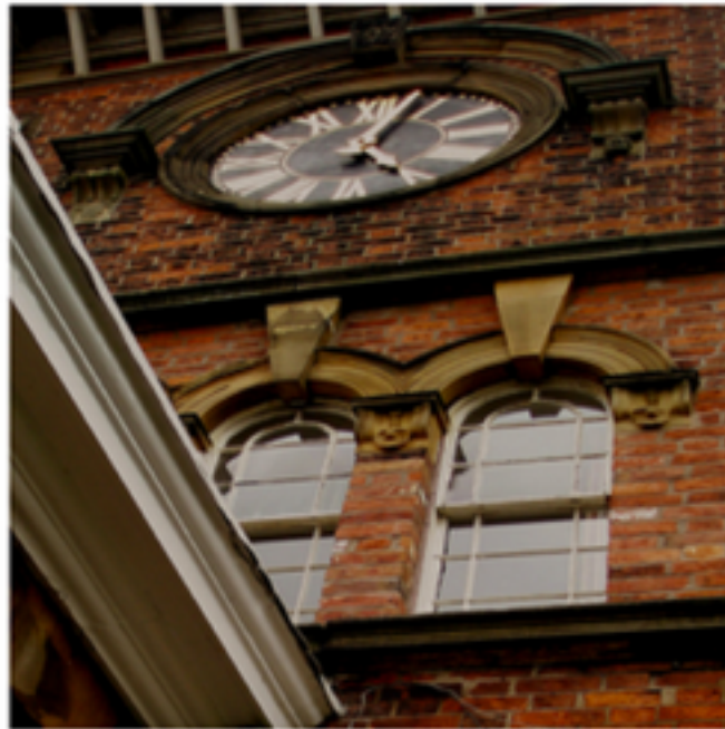
A large clock mounted to the side of a building.
