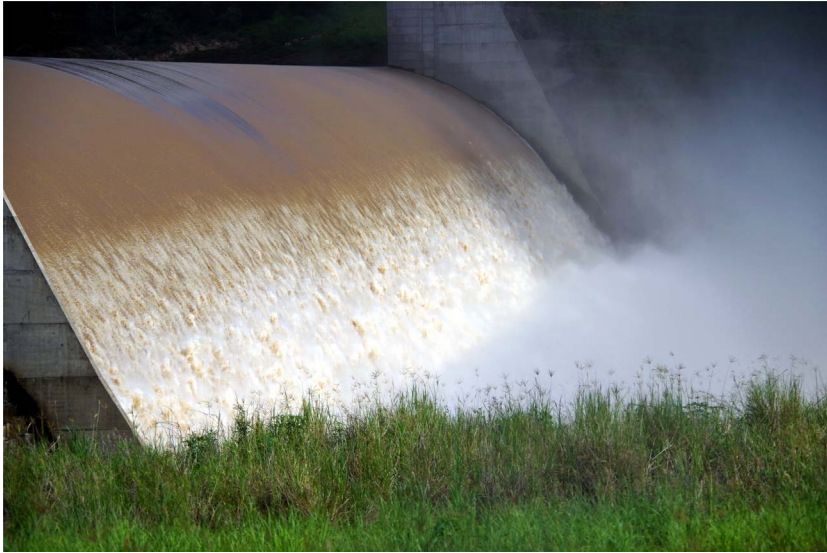
Fig. 1. Prototype stepped spillway: Paradise dam's (Australia) operation on 5 March 2013 - Q = 2300 \text{ m}^3/\text{s} , Re = 7.3 \times 10^6 , h = 0.62 \text{ m} - The location of the inception point of free-surface aeration is clearly seen.
