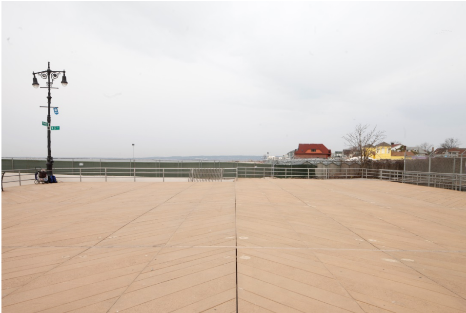
Coney Island (Riegelmann) Boardwalk , west end at West 37th Street Sarah Moses (LPC), 2018
