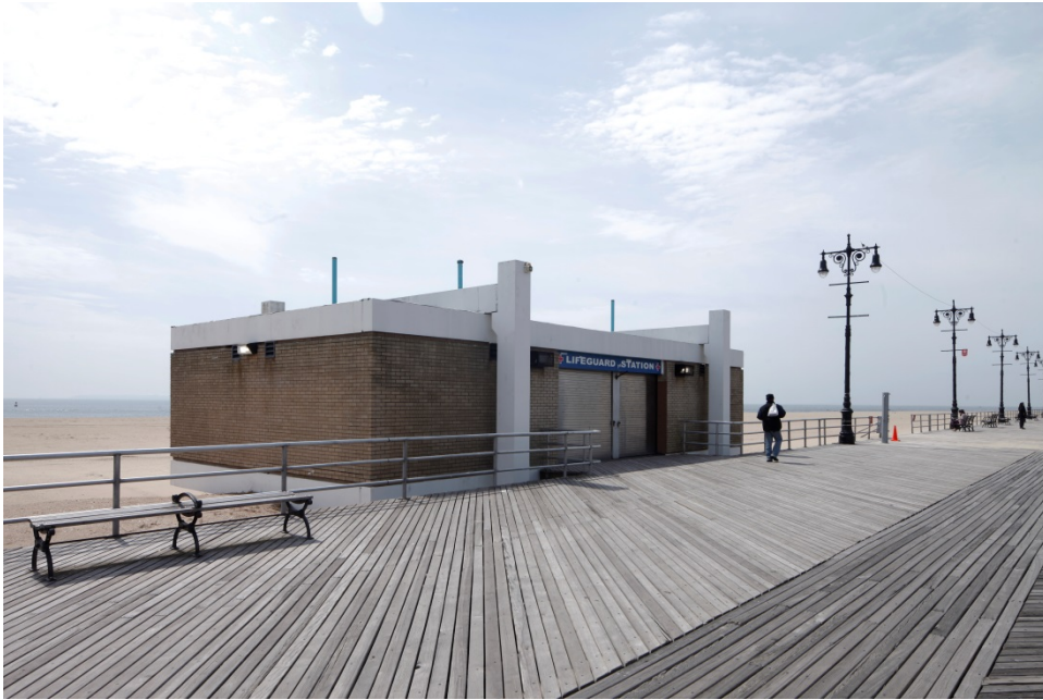
Coney Island (Riegelmann) Boardwalk , lifeguard station near West 22nd Street Sarah Moses (LPC), 2018
