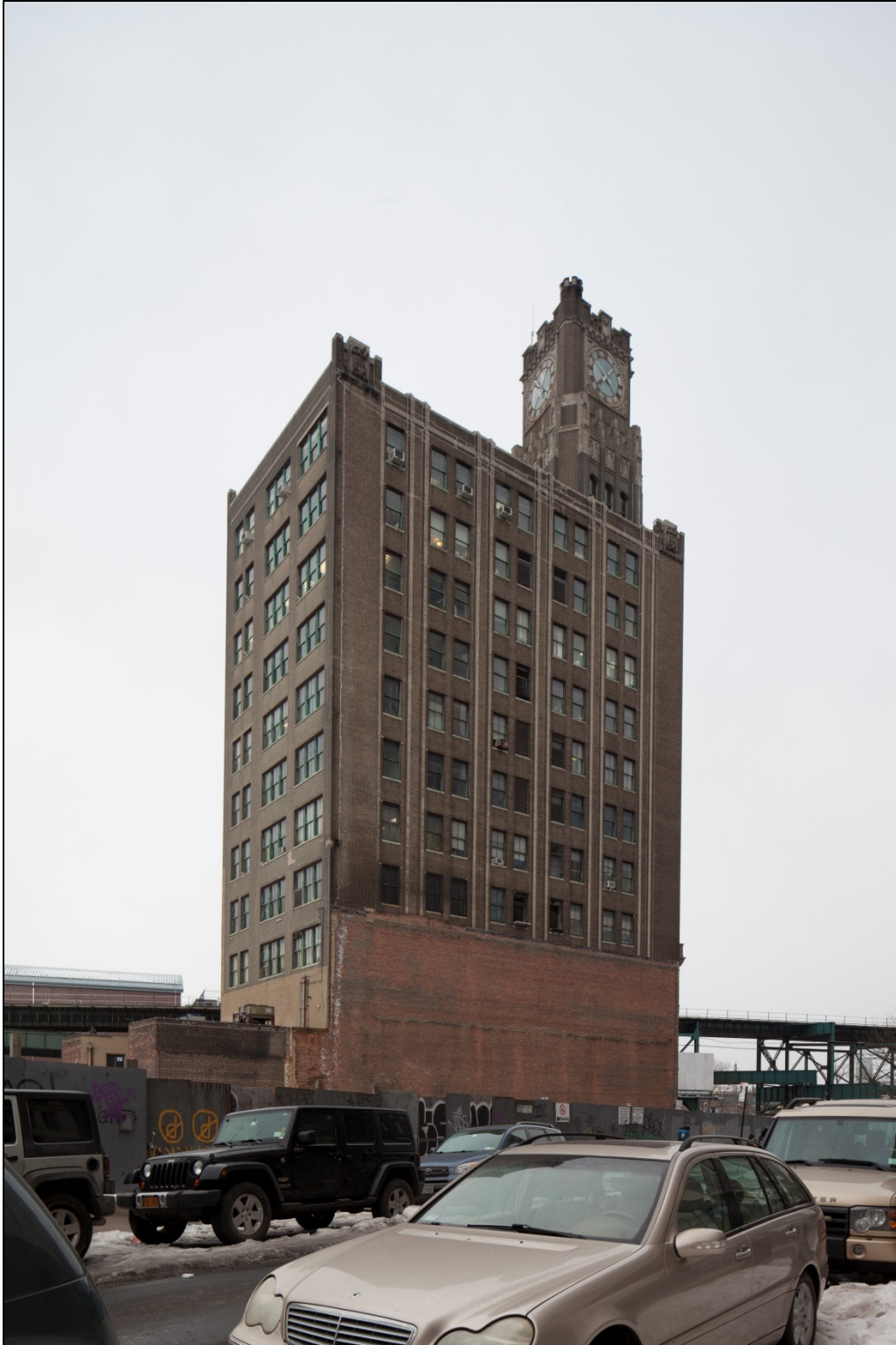
Bank of the Manhattan Company Building, Long Island City West and north facades
