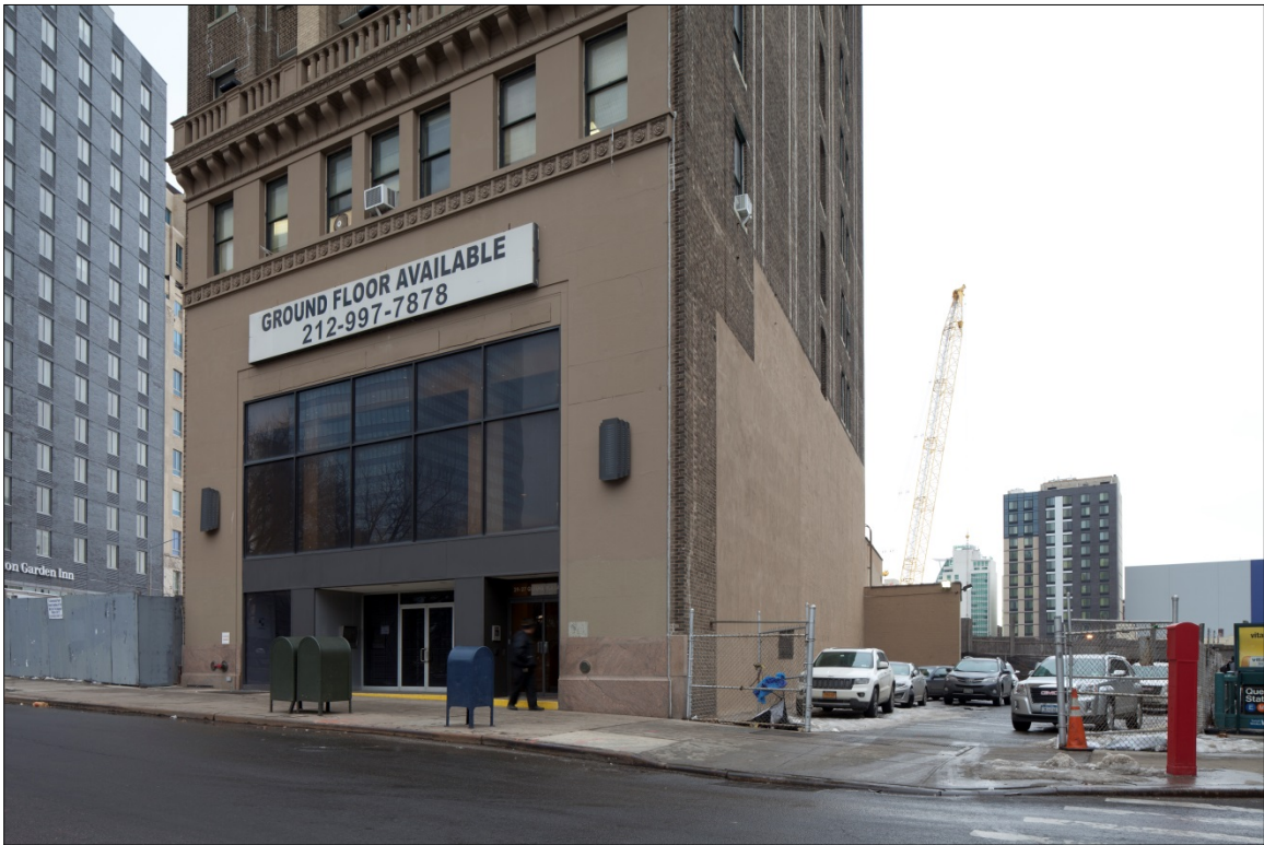
Bank of the Manhattan Company, Long Island City Photos by Matthew A. Postal (clock) and Christopher D. Brazee (base), 2015
