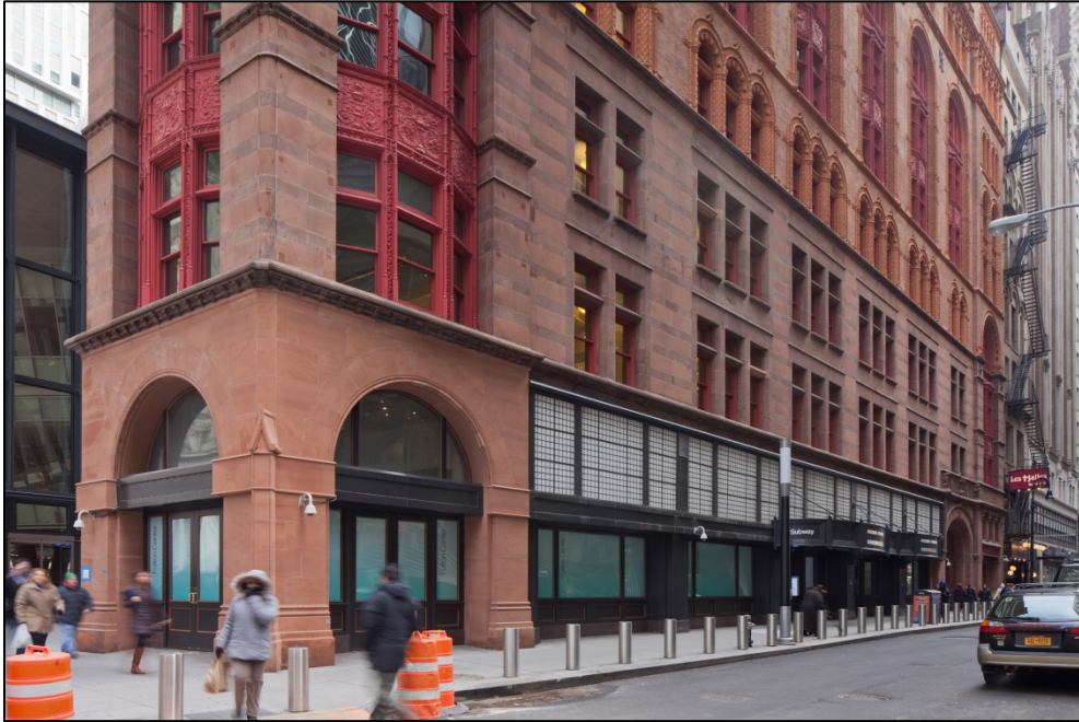
Corbin Building, John Street (South) Elevation (entrance detail) Photo: Christopher D. Brazee (2015)
