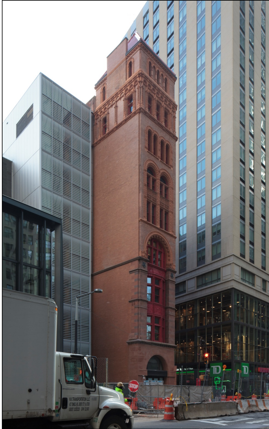
Corbin Building, Broadway (West) Elevation Photo: Christopher D. Brazee (2015)
