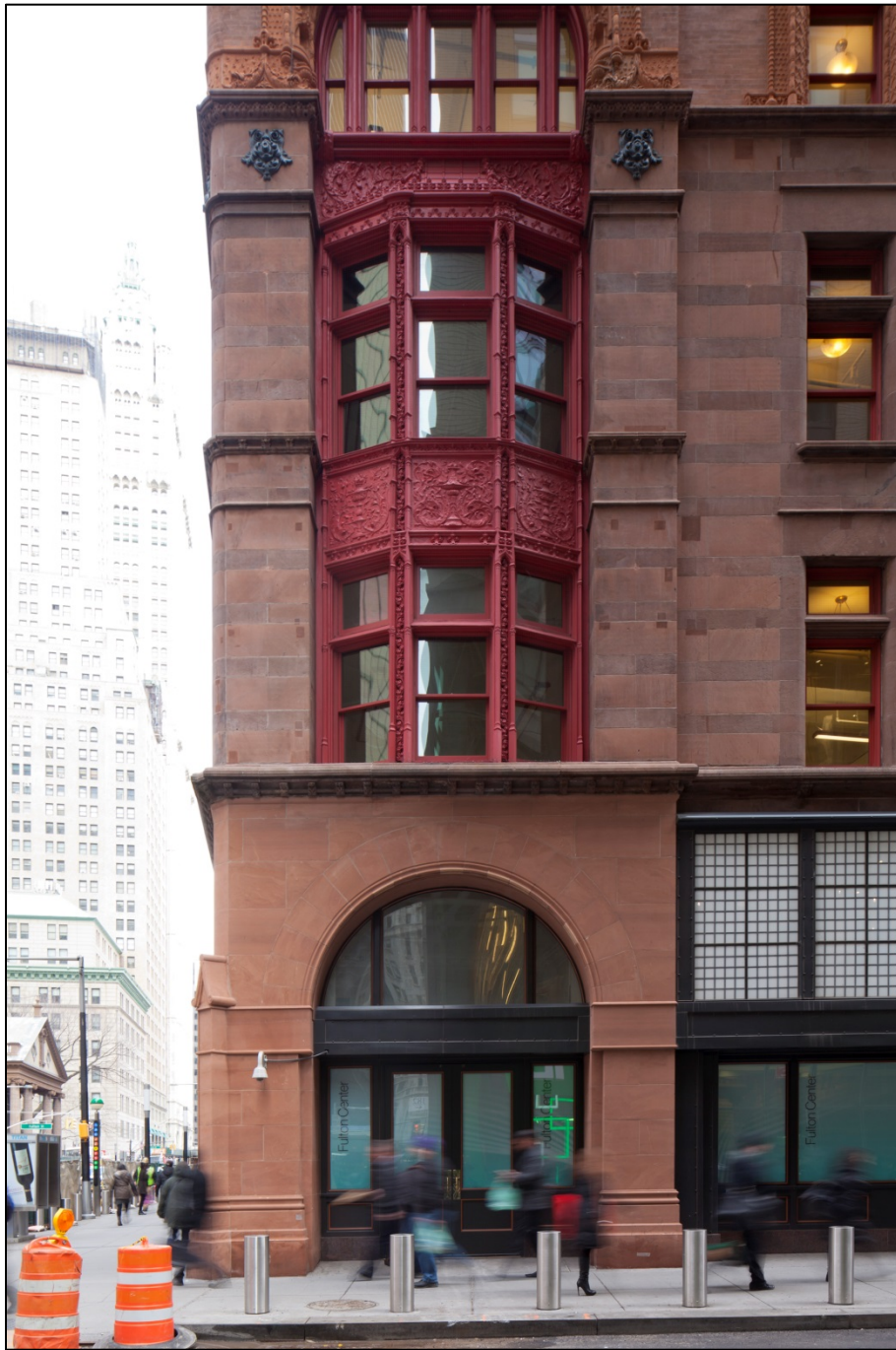
Corbin Building, John Street (South) Elevation (entrance detail) Photo: Christopher D. Brazee (2015)
