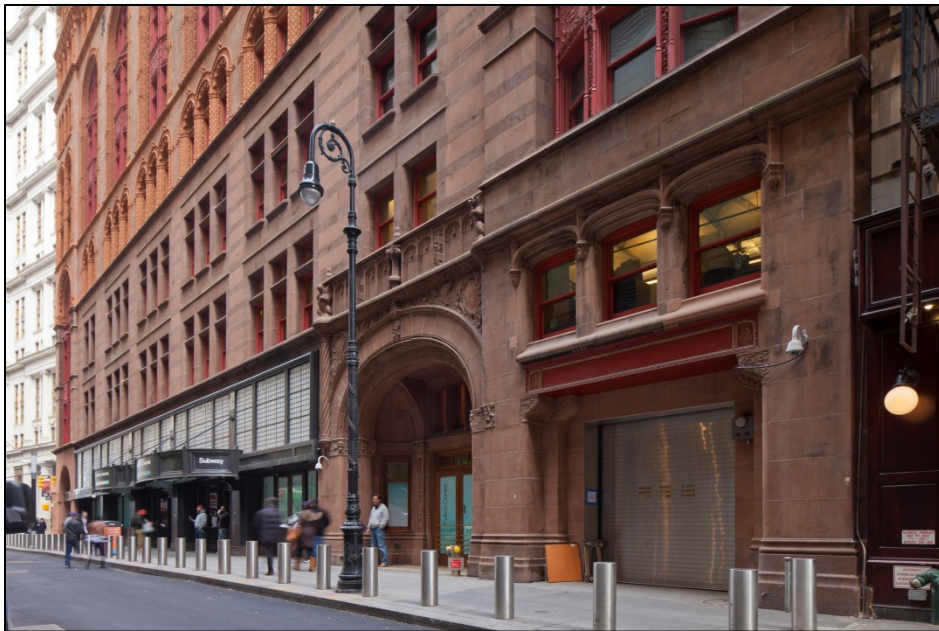
Corbin Building, John Street (South) Elevation (looking west) Photo: Christopher D. Brazee (2015)
