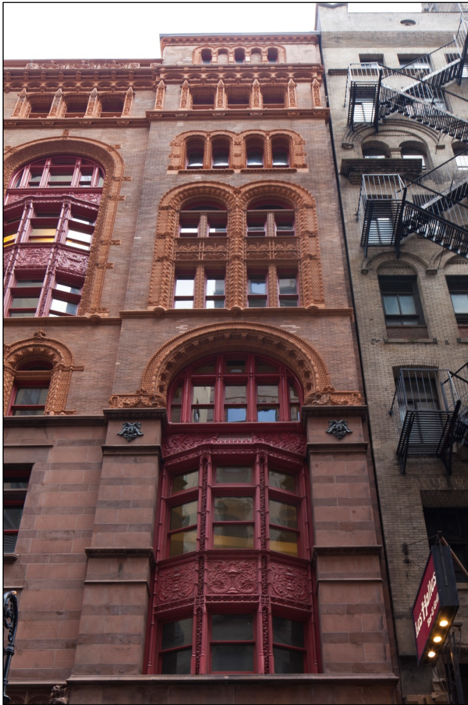
Corbin Building, John Street (South) Elevation (details) Photo: Christopher D. Brazee (2015)
