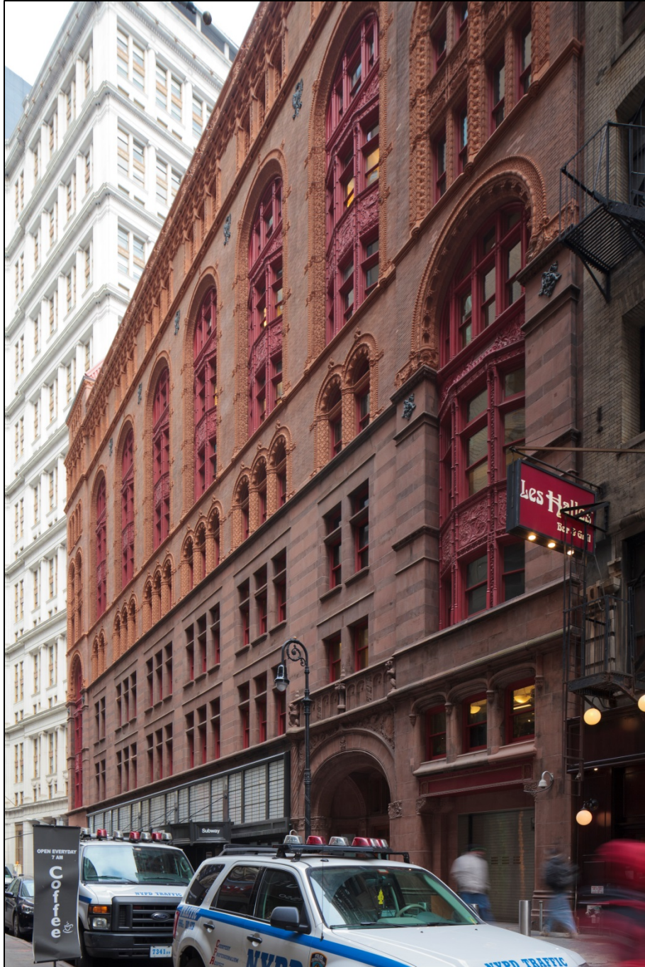
Corbin Building, John Street (South) Elevation Photo: Christopher D. Brazee (2015)
