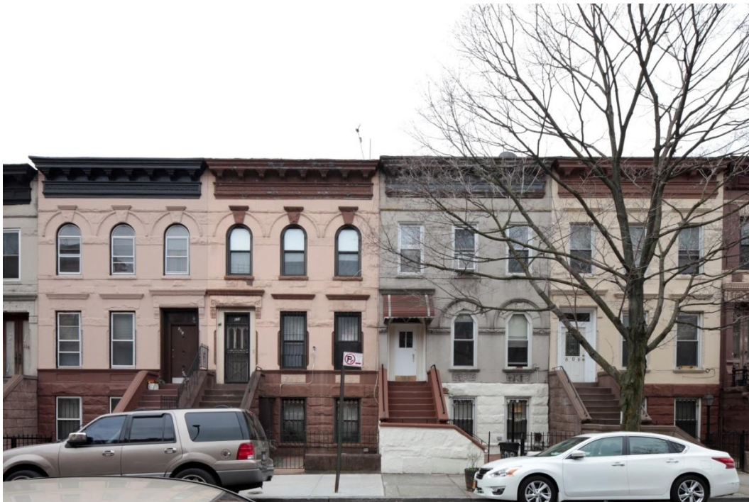
606 to 614 A Halsey Street (1897, Hugo Smith, architect): Some rows were designed in a combination of styles, such as this group of two-family houses that features Romanesque- and Renaissance-inspired ornament. Photo: Christopher D. Brazee, 2013
