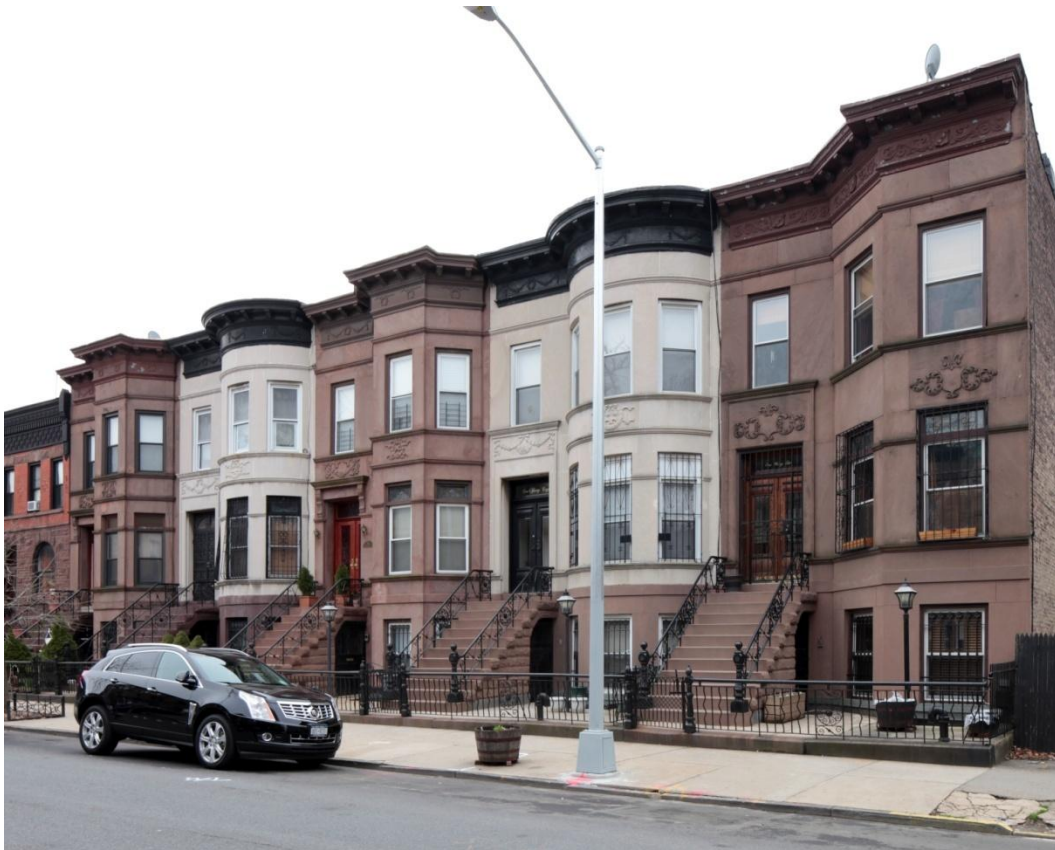
146 to 154 Bainbridge Street (1898, Walter F. Clayton, architect): These well-preserved, Renaissance Revival style houses feature full-height projecting bays, alternating between curved and angled, and a variety of carved classical ornament, such as swags, shields, moldings, and brackets, that unifies the row. Photo: Christopher D. Brazee, 2013
