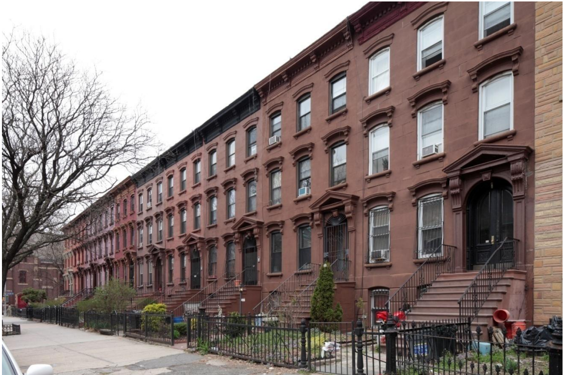
267 to 287 Macon Street , built in 1872-73, display typical characteristics of Italianate style row houses, such as pedimented door hoods supported by large scrolled brackets, segmentally-arched window openings with molded and bracketed lintels, and projecting cornices with frieze panels and dentils. Photo: Christopher D. Brazee, 2013
