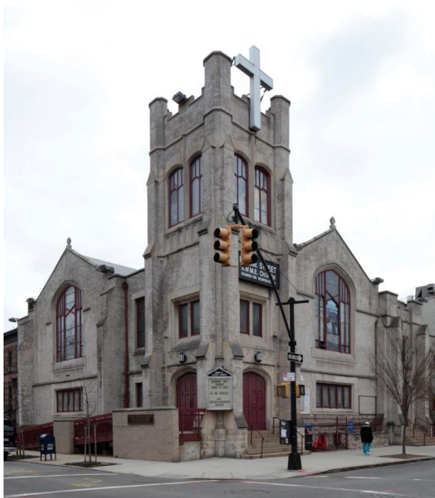
Grace Presbyterian Church (now the Bridge Street African Wesleyan Methodist Episcopal Church) 279 Stuyvesant Avenue (aka 634-640 Jefferson Avenue): Originally built in 1890, it was enlarged and given this new Gothic Revival style façade, designed by the architectural firm Leeming & Kirk, in 1907. Photo: Christopher D. Brazee, 2013
