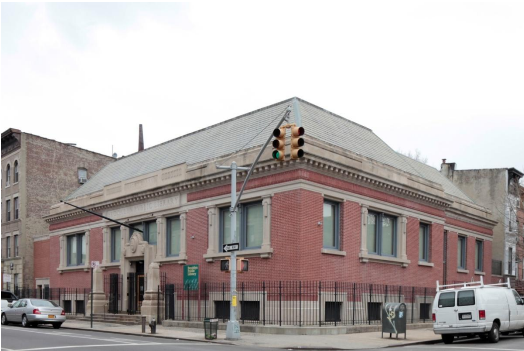
Brooklyn Public Library, Macon Branch, 361 Lewis Avenue (aka 361-371 Lewis Avenue; 417-425 Macon Street) : Designed by Richard A. Walker of the architectural firm Walker & Morris, this Beaux Arts style building, completed in 1907, features Flemish bond, cheek walls terminating in obelisks, limestone door and window surrounds with stylized pilasters, and a brick frieze with a plaque carved with Brooklyn Public Library. Photo: Christopher D. Brazee, 2013
