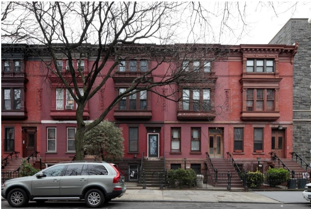
278 to 290 Macon Street (1888, Thomas F. Houghton, architect): This row displays many typical Queen Anne style characteristics, such as rough-faced stonework, metal-clad oriels featuring classical details, foliated panels, and bracketed cornices decorated with dentils, rosettes, and angular panels. Photo: Christopher D. Brazee, 2013
