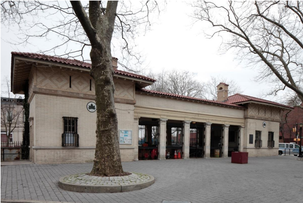
Fulton Park Comfort Station (1908, Helmle & Huberty, architects): Designed in the Mediterranean Revival, this prominent park building features an open arcade, brick diaperwork, end pavilions, decorative cupolas, exposed wood rafters, and a Spanish tile roof. Photo: Christopher D. Brazee, 2013
