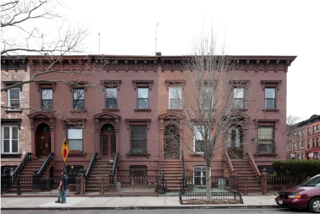
284 to 288 Stuyvesant Avenue (1880-81, James P. Miller, builder): an exceptionally-intact row of neo-Grec style row houses, featuring heavy main-entrance surrounds with incised fluting, large, angular brackets, and triangular pediments, as well as cast-iron newel posts on the stoops. Photo: Christopher D. Brazee, 2013
