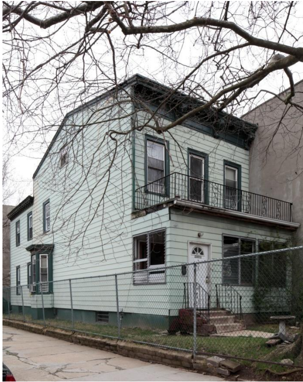
329 Stuyvesant Avenue , a freestanding, Italianate Style house (with alterations) probably built during Bedford-Stuyvesant's early period of suburbanization in the mid-19 th century. Photo: Christopher D. Brazee, 2013
