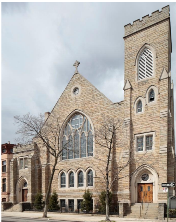
The Herkimer Street Baptist Church (now the Bethany Baptist Church) 456 Marcus Garvey Boulevard (aka 141-147 Decatur Street and 218-220 Macdonough Street) , built in 1888 to the designs of Albert V. Porter, is faced in stone and features typical Gothic Revival style elements, such as pointed arch fenestration with ribbed sash, gabled buttresses, and a crenellated tower. Photo: Christopher D. Brazee, 2013
