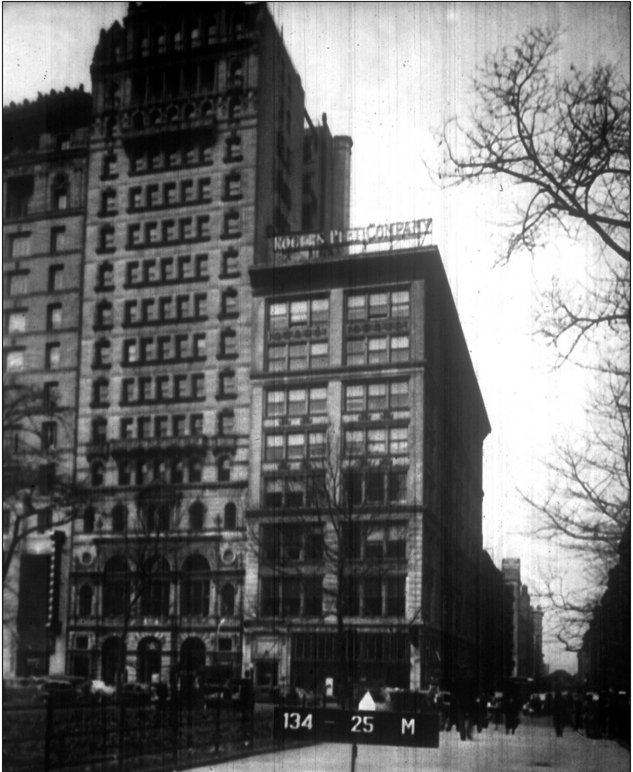
Rogers, Peet & Company Building Photo: New York City Department of Taxes (c. 1939) Courtesy New York City Municipal Archives
