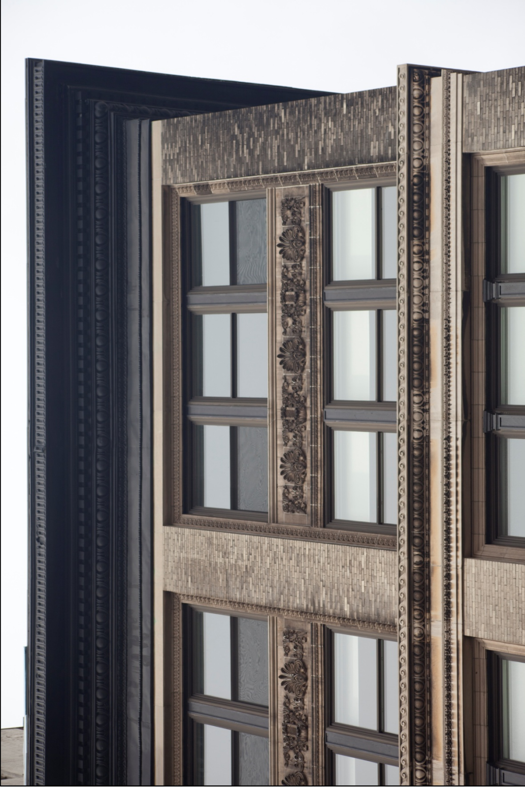
Rogers, Peet & Company Building Detail of terra-cotta spandrel and molded cornice Photo: Christopher D. Brazeel, 2010
