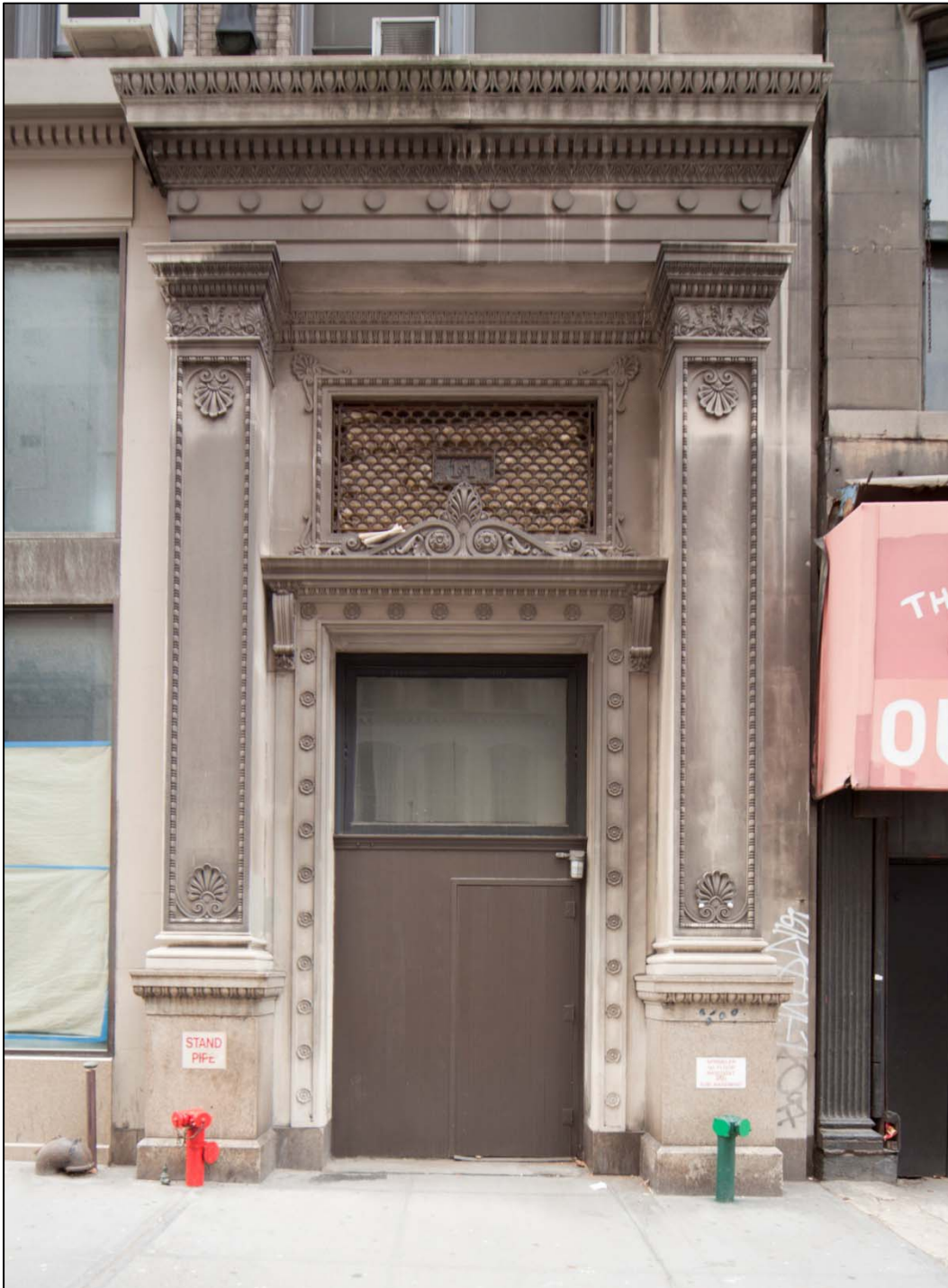
Rogers, Peet & Company Building Stone entablature framing Warren Street entrance Photo: Christopher D. Brazee, 2010
