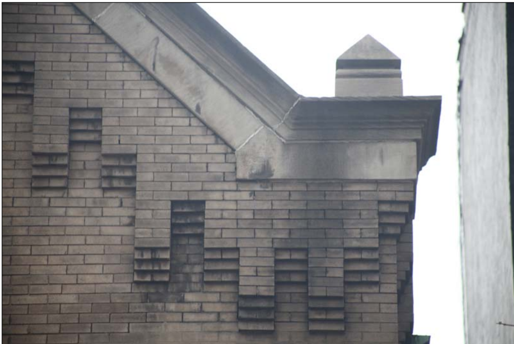
Corbels and finial
