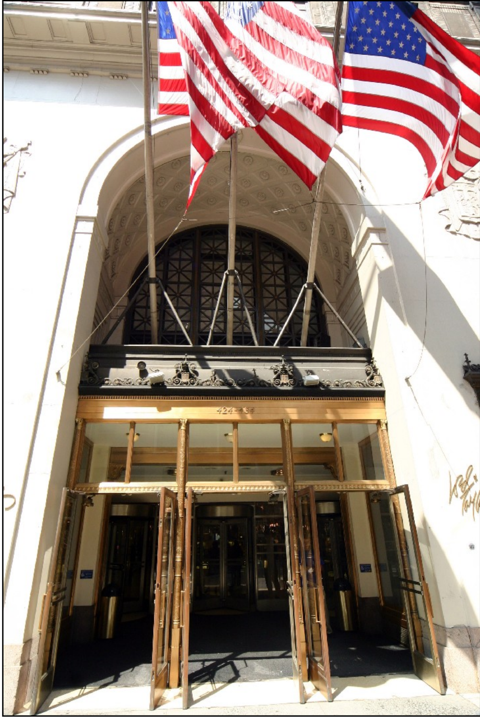
Lord & Taylor Building, Fifth Avenue entrance
