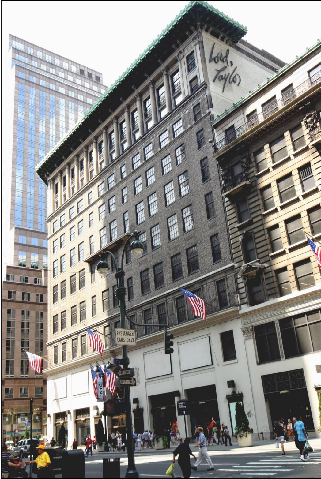
Lord & Taylor Building , view from the northeast Photo: Carl Forster
