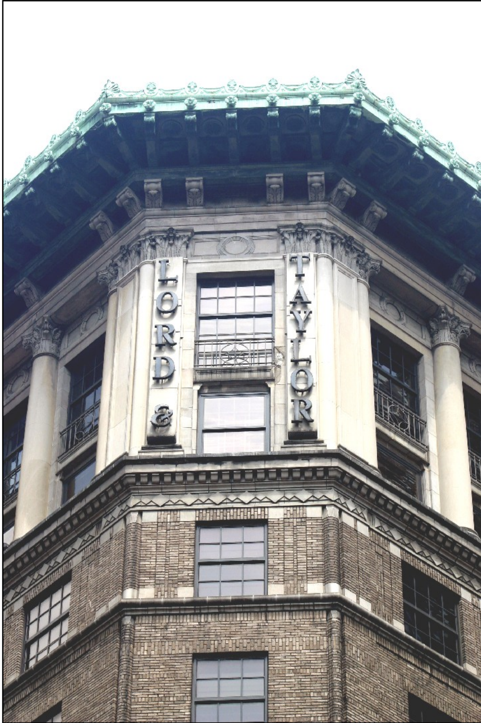
Lord & Taylor Building , chamfered corner, detail Photo: Carl Forster
