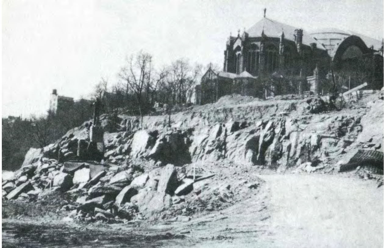
Catskill Aqueduct Pumping Station, Morningside Park (1916) Source: American Scenic and Historic Preservation Society
