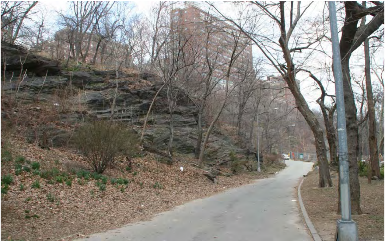
Morningside Park, Rockwork, Stairs, and Path Near 112th Street
