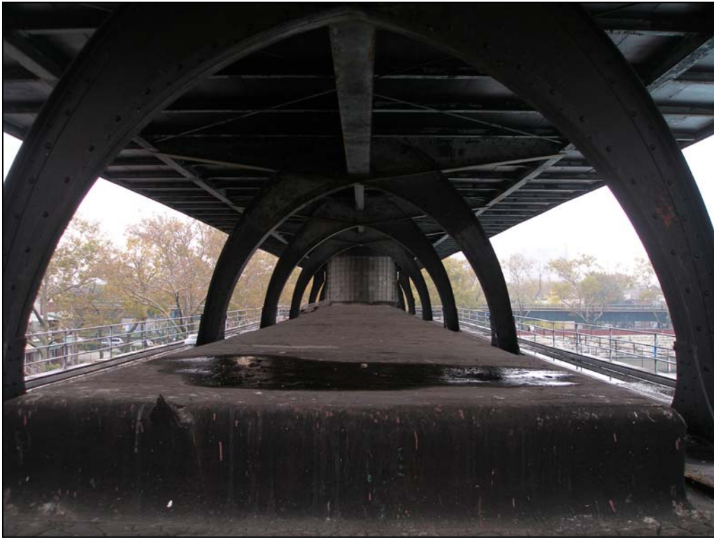
Betsy Head Play Center Parabolic arches, roof canopy and roof deck Photo: Christopher D. Brazee, 2007
