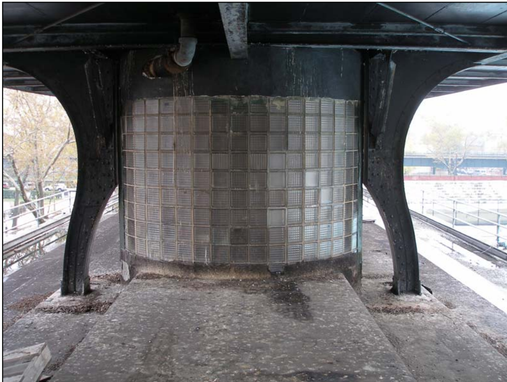
Betsy Head Play Center Detail of glass block lighting feature on roof deck Photo: Christopher D. Brazee, 2007
