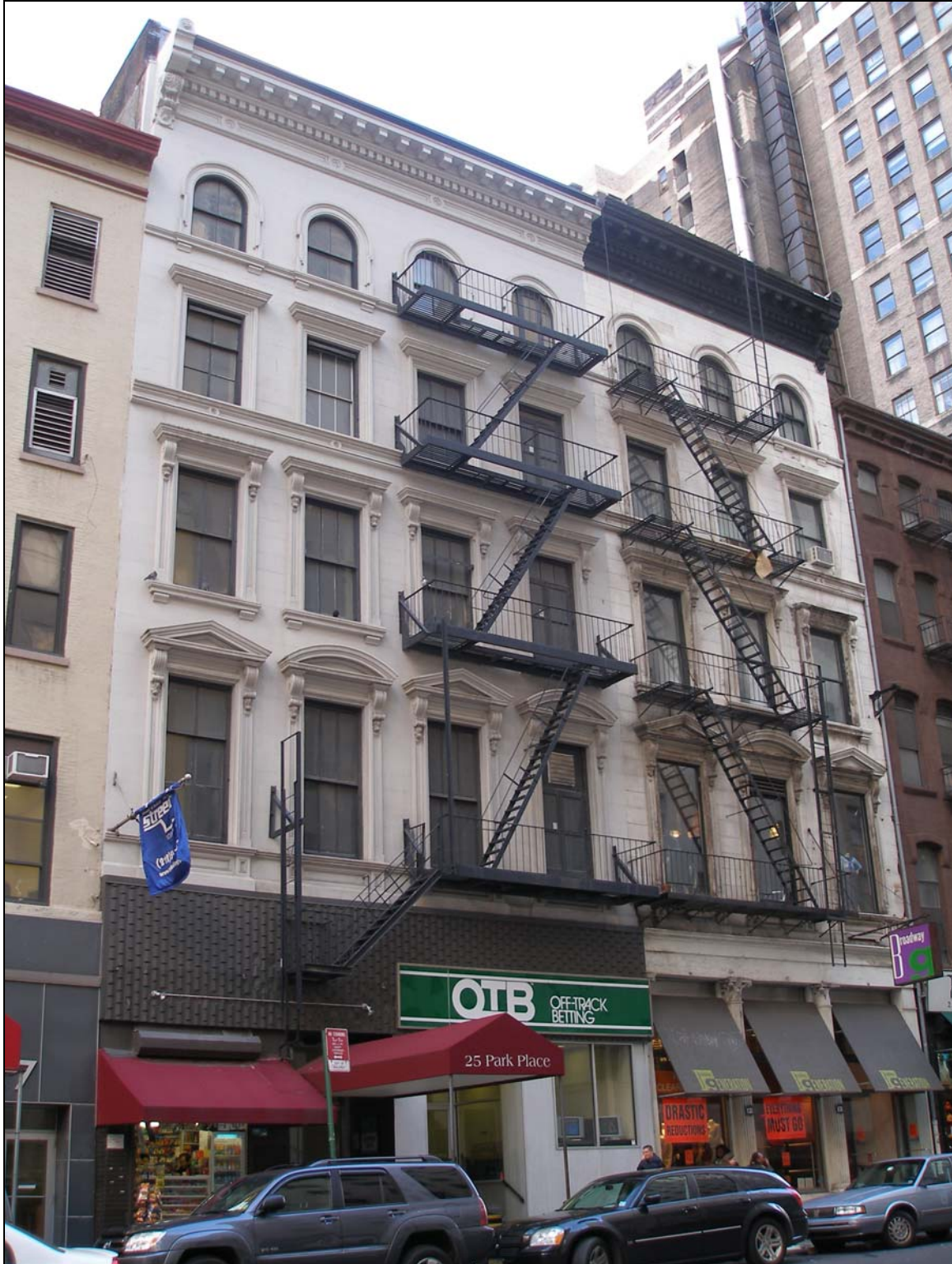
25 and 23 Park Place Buildings, Park Place elevations Photo: Amanda Davis
