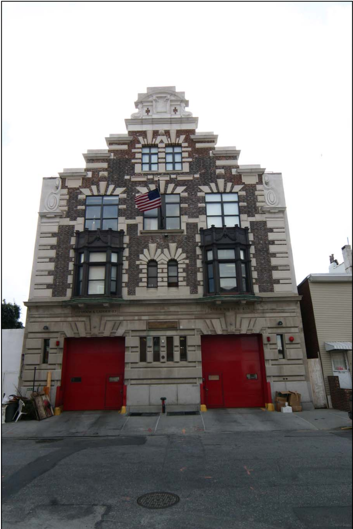
Fire Engine Company No. 258, Hook and Ladder Company No. 115 10-40 47th Avenue (aka 10-38 to 10-40 47th Avenue) Queens
