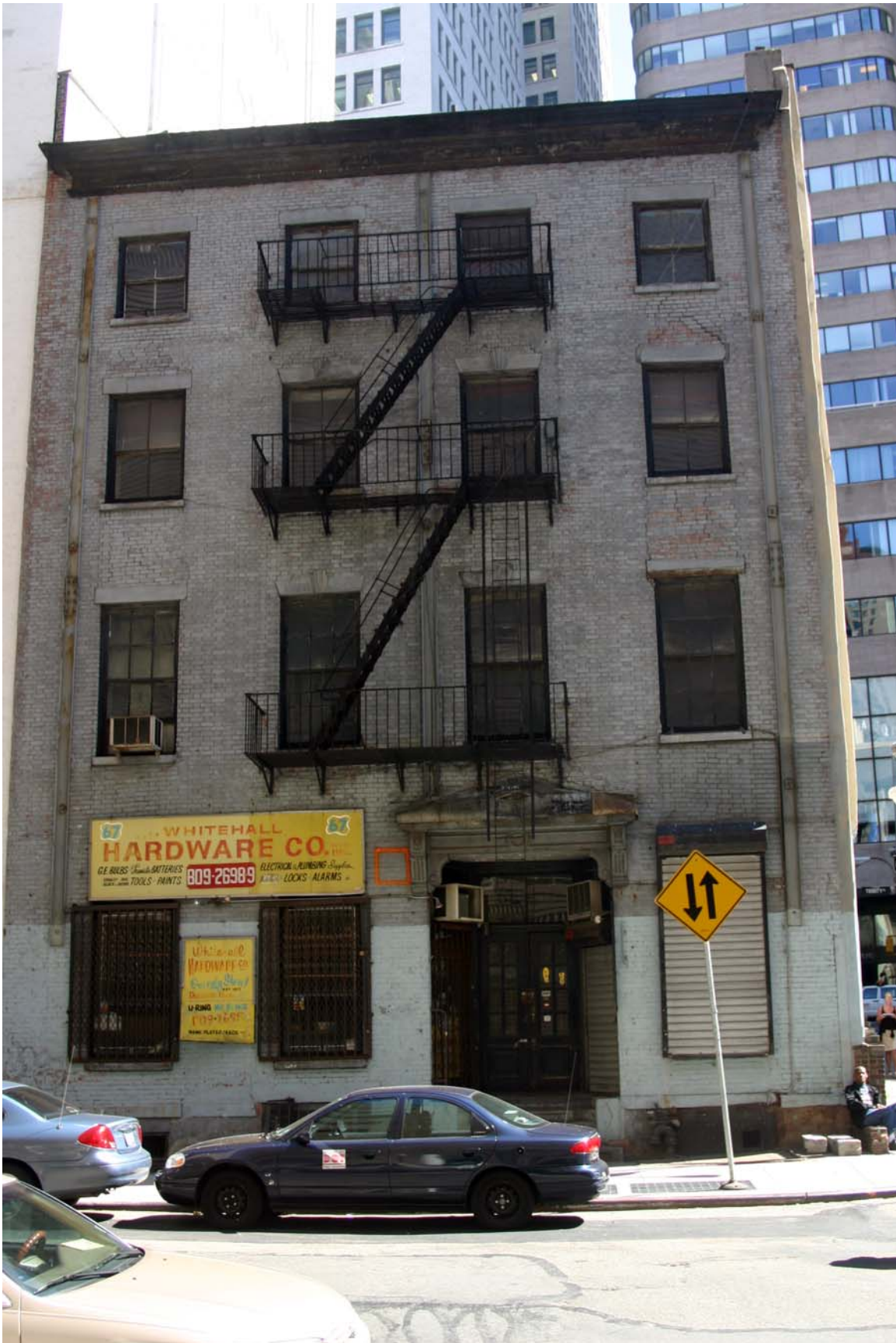
Robert and Anne Dickey House, front façade Photo: Carl Forster, LPC
