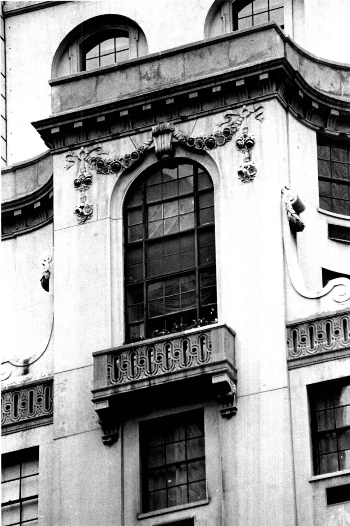
Aeolian Building (later Elizabeth Arden Building), detail of Fifth Avenue facade Photo: Carl Forster
