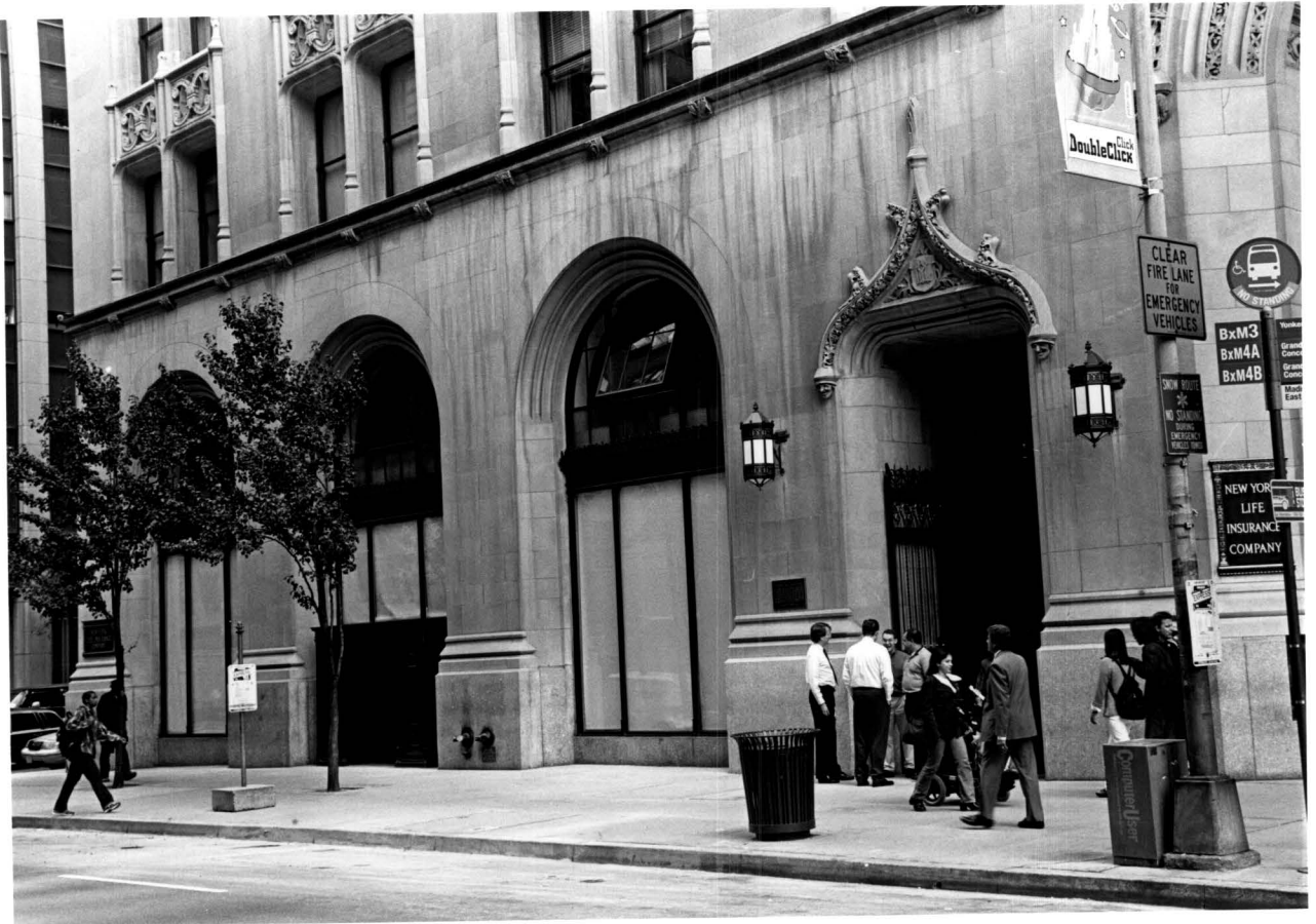
Madison Avenue facade at the ground floor and mezzanine.
