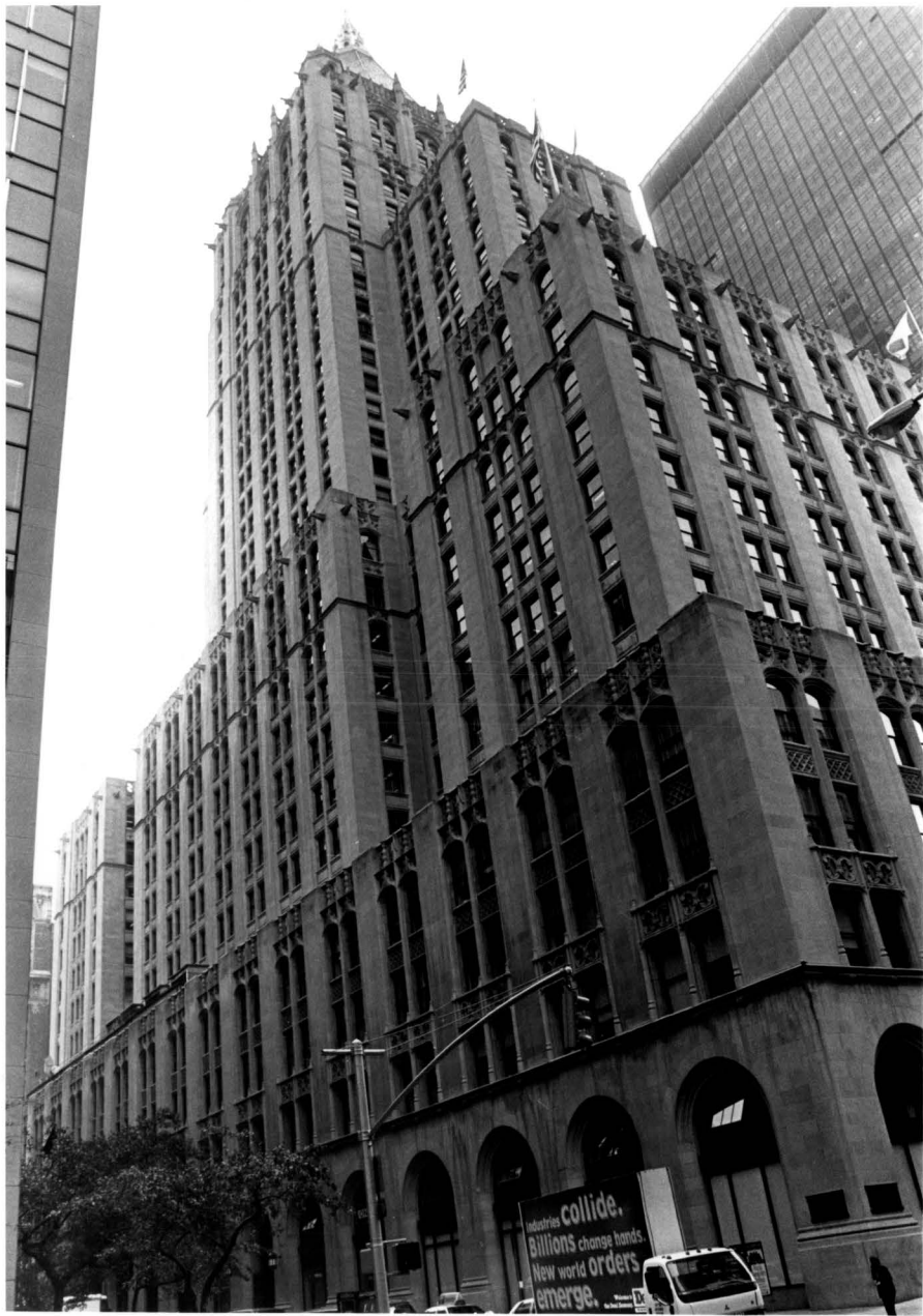
East 27 th Street facade.
