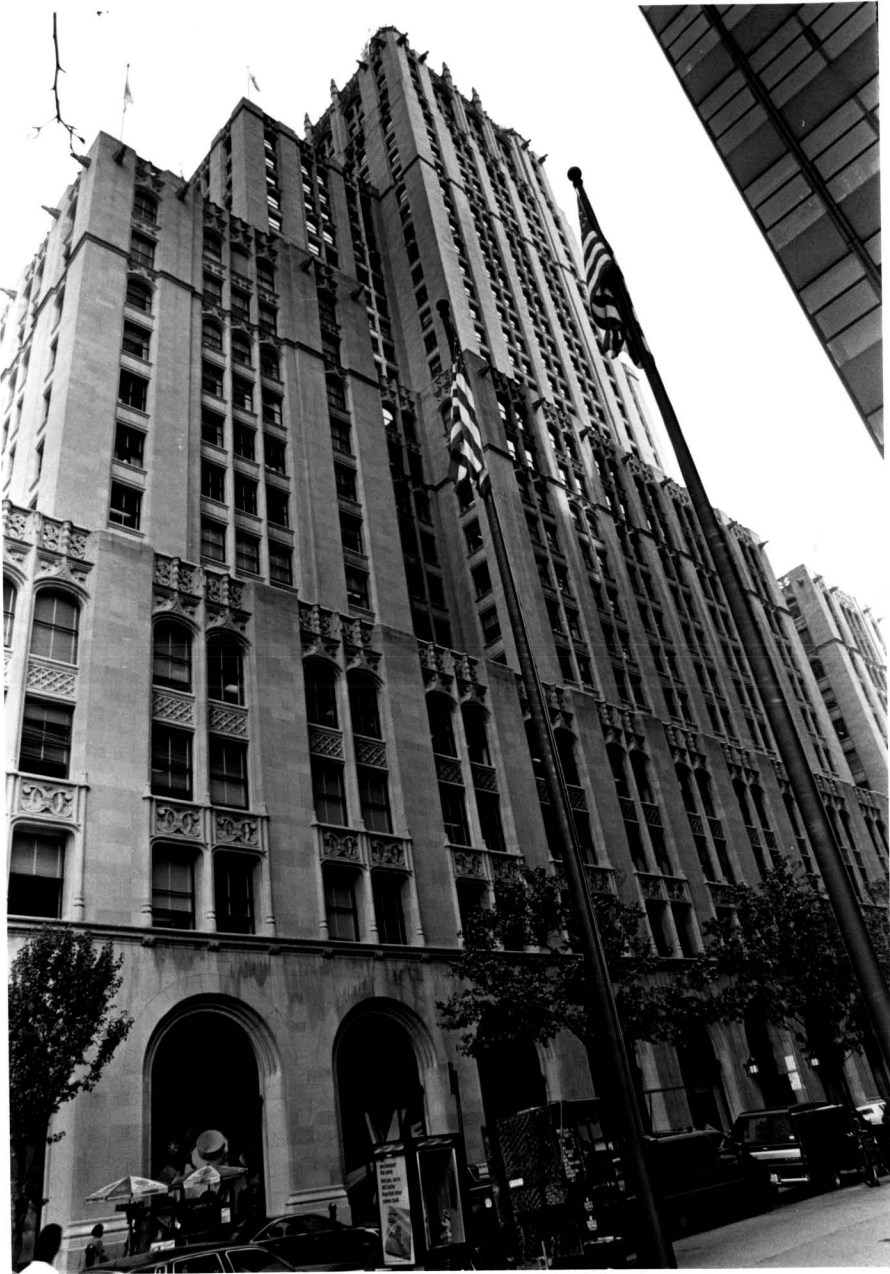
East 26 th Street facade.
