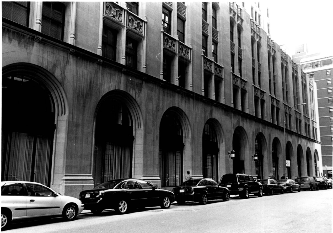
East 26 th Street facade.
