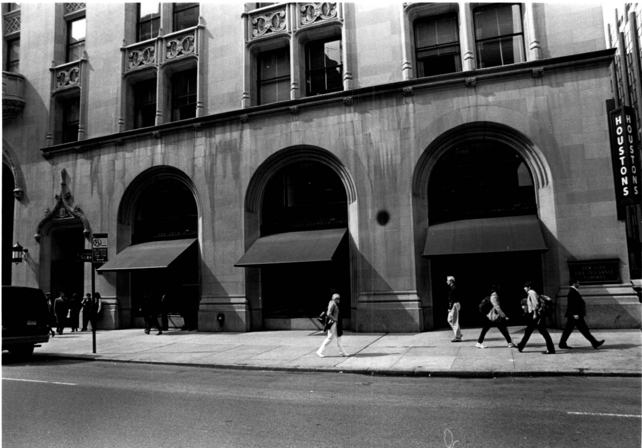
Park Avenue South facade at the ground floor and mezzanine.
