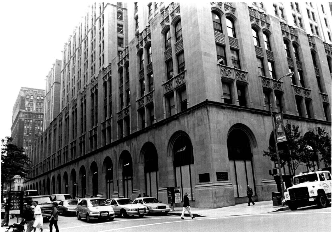
East 27 th Street facade.
