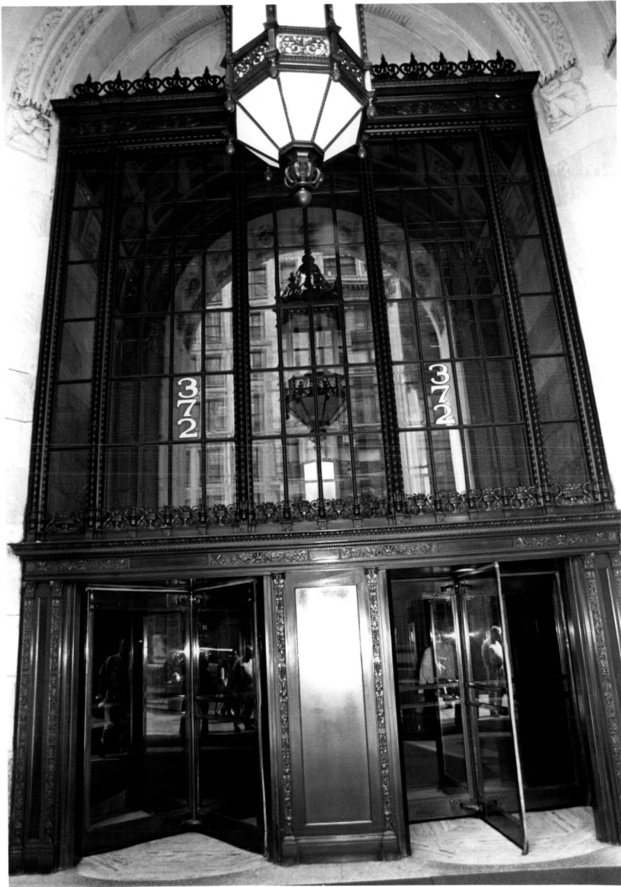
Entryway from Park Avenue South vestibule to lobby. Photo: Carl Forster, LPC, 2000.
