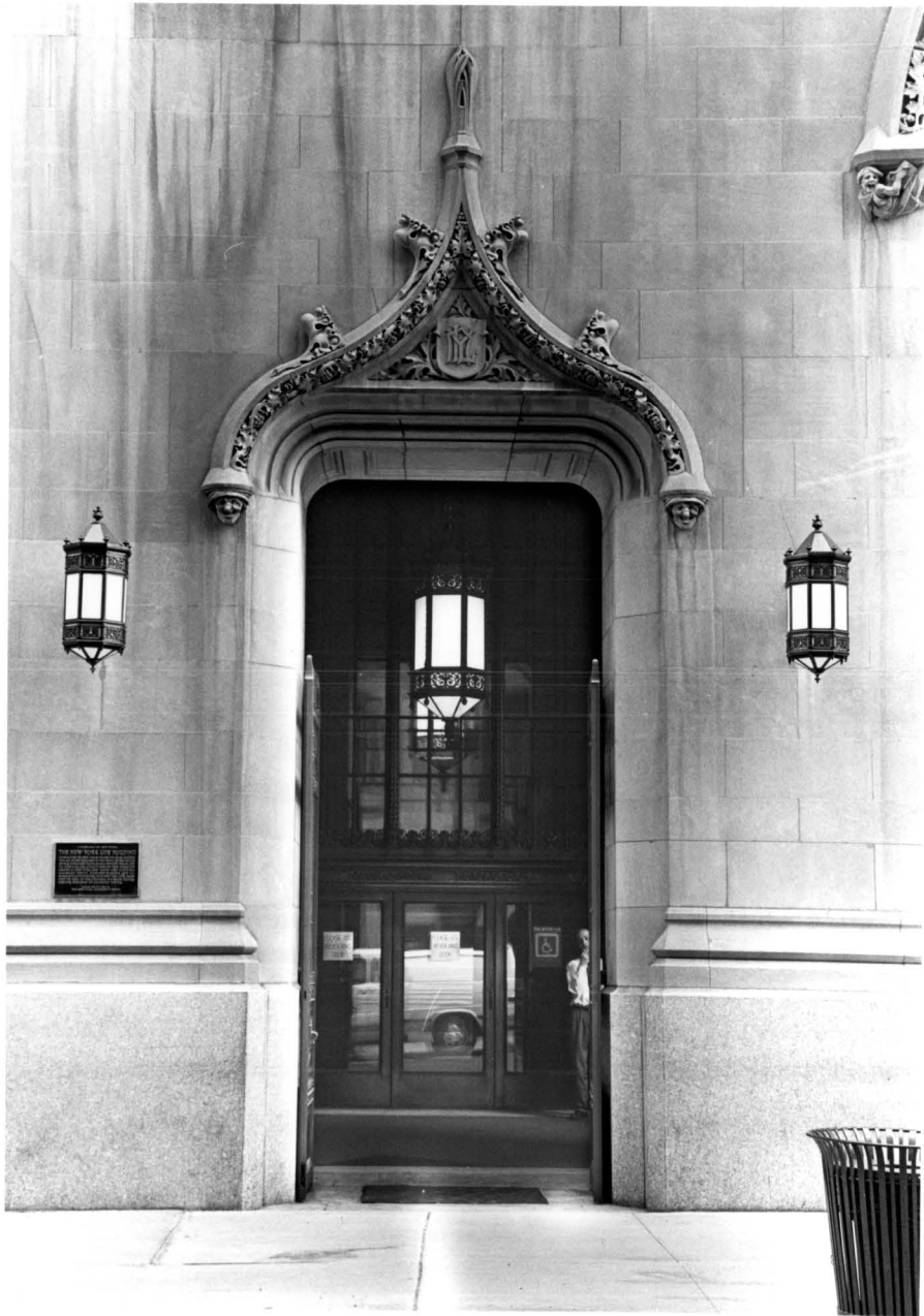
Side entrance to outer vestibule facing Madison Avenue. Photo: Carl Forster, LPC, 2000.
