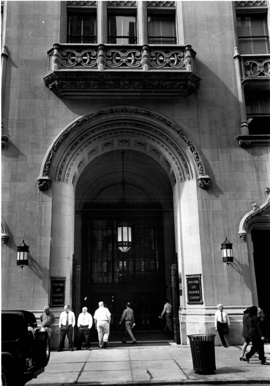
Main entryway to outer vestibule facing Park Avenue South. Photo: Carl Forster, LPC, 2000.
