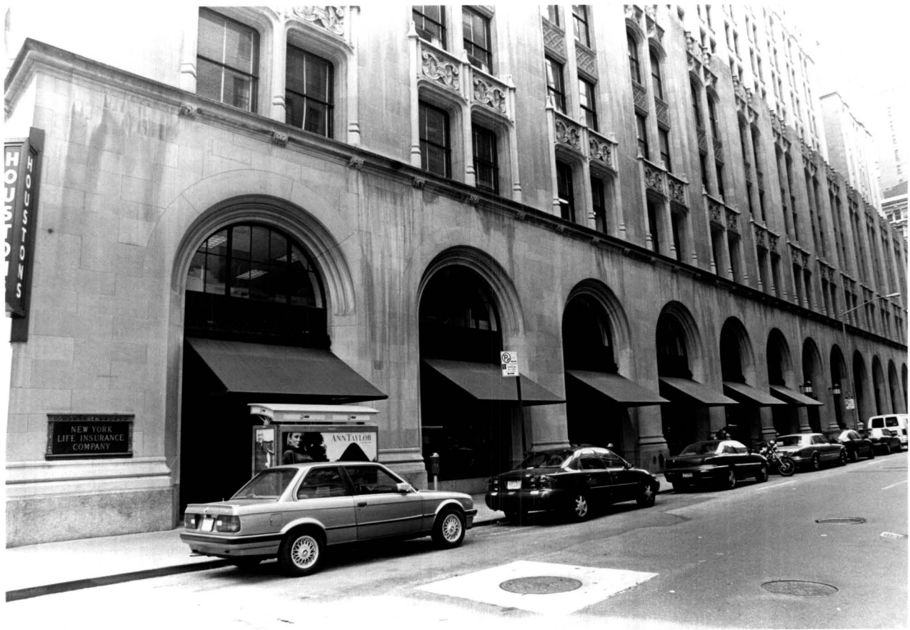
East 27 th Street facade.
