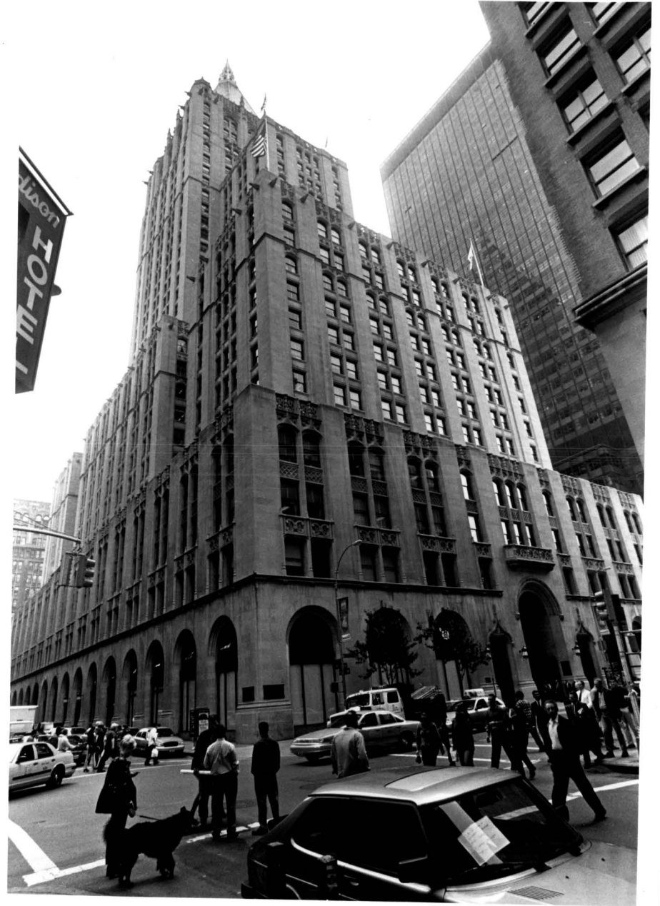
Madison Avenue facade.
