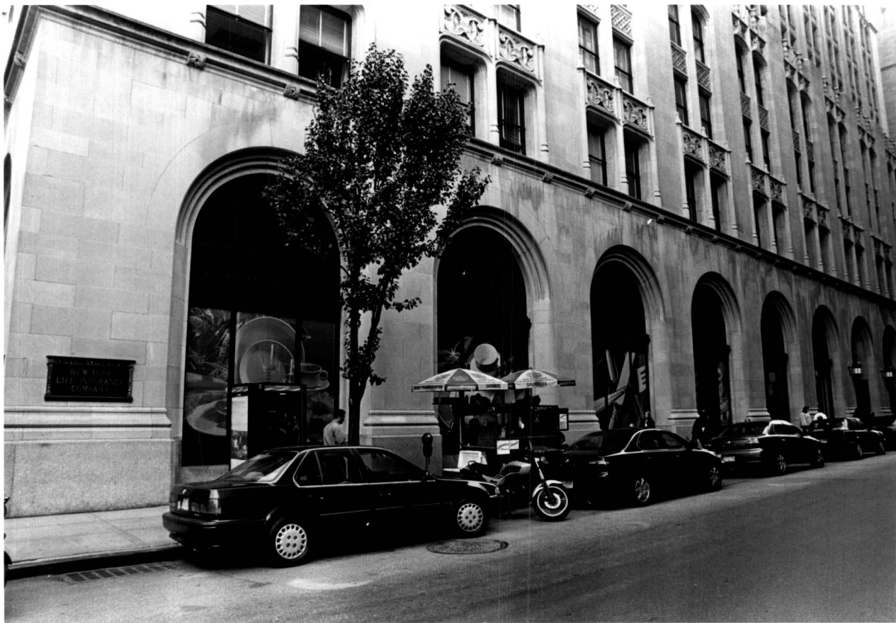
East 26 th Street facade.
