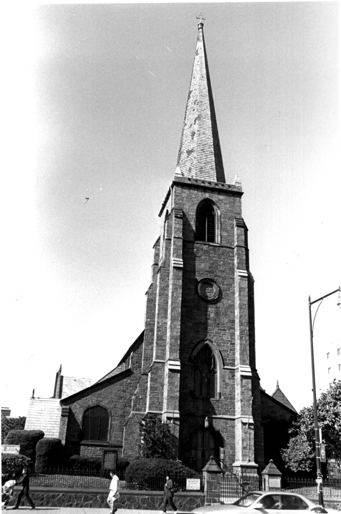
St. George's (Episcopal) Church 38-02 Main Street, Flushing Queens Photo: Carl Forster
