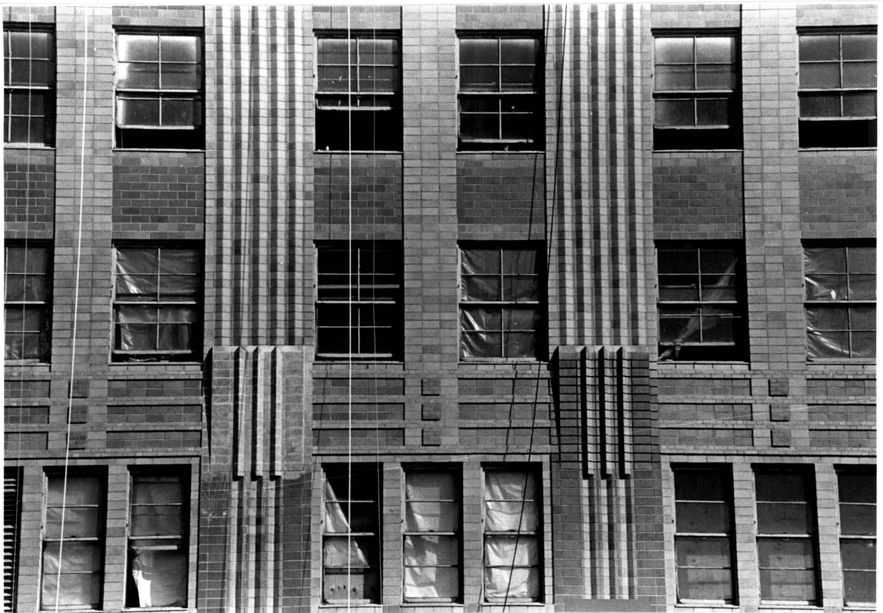
21 West Street, Manhattan Facade Details Photos: Carl Forster
