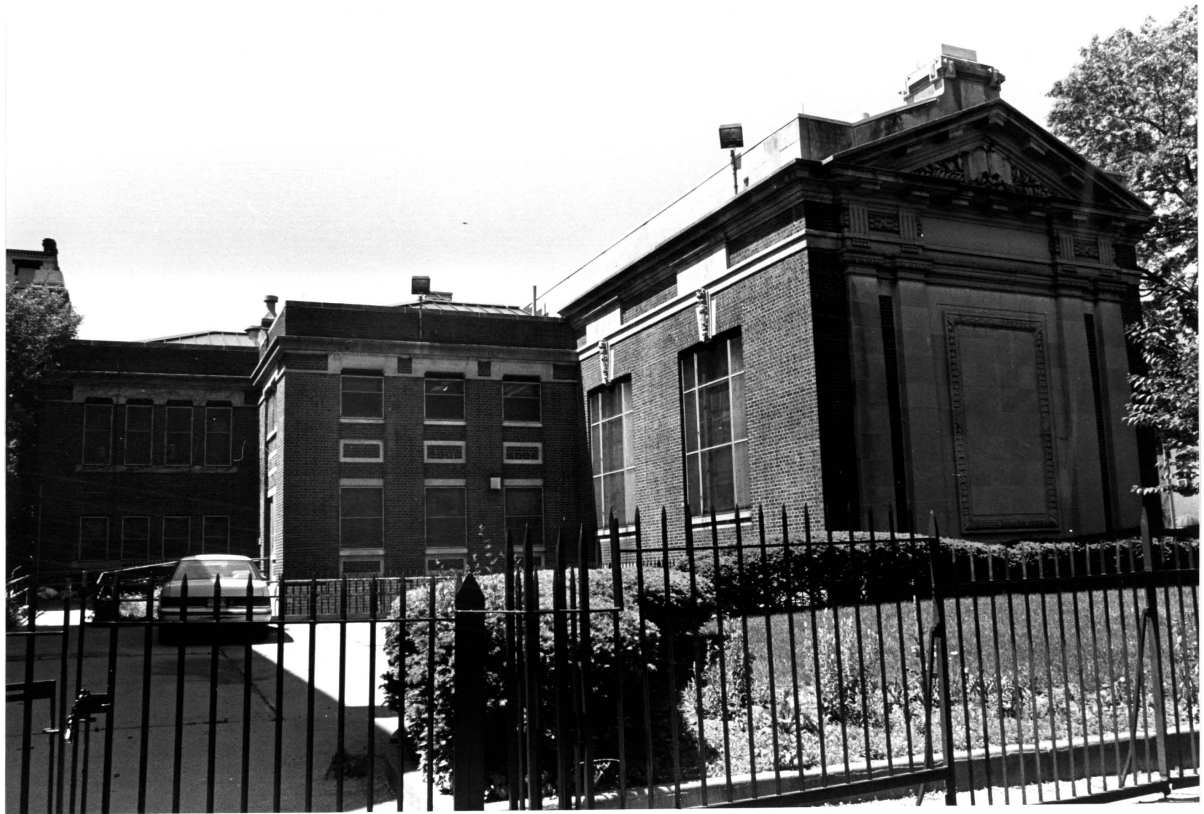
Brooklyn Public Library, Park Slope Branch, 431 Sixth Avenue, Brooklyn Eighth Street elevation Photo: Carl Forster
