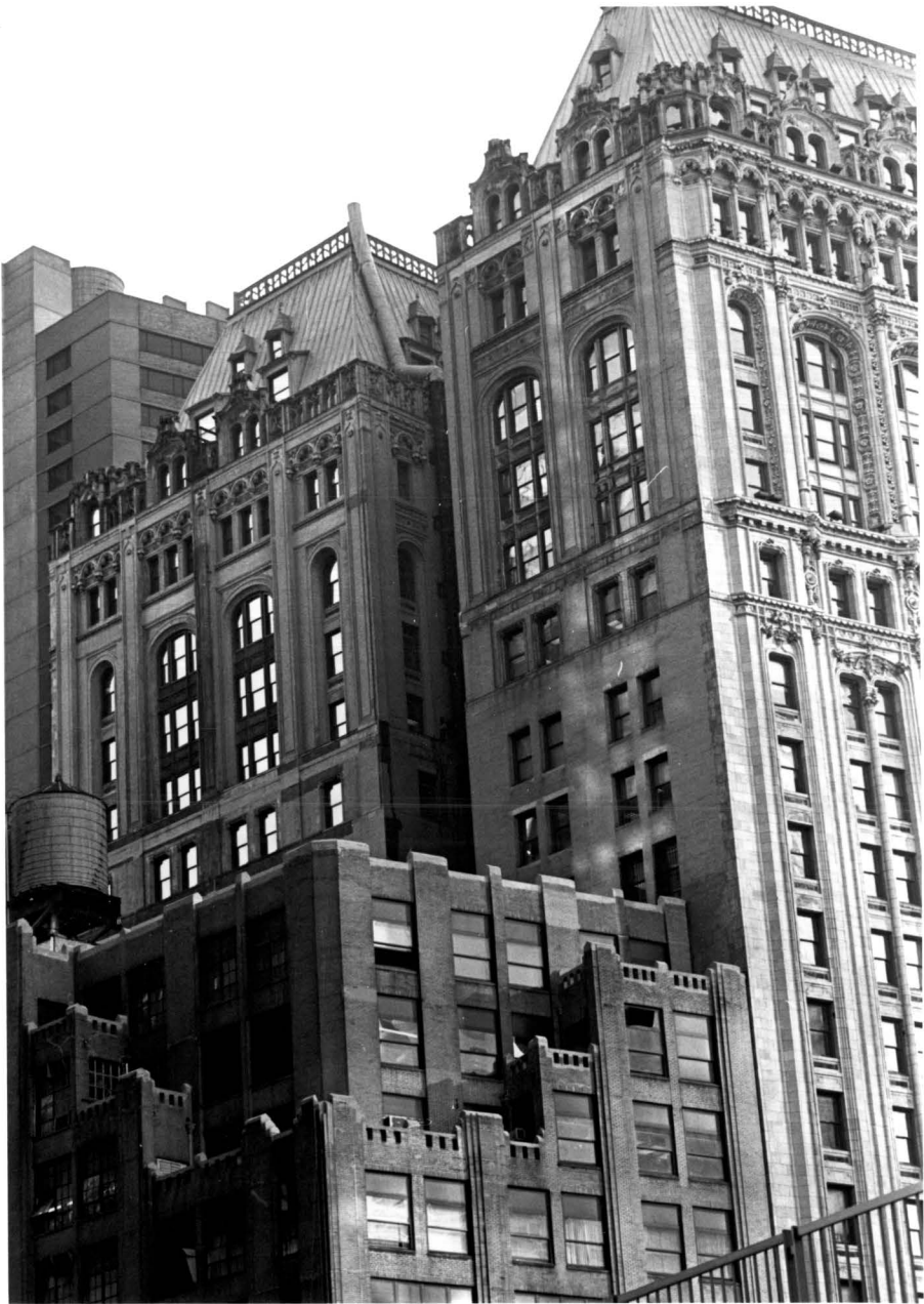
Eastern elevation at upper stories of West Street Building
