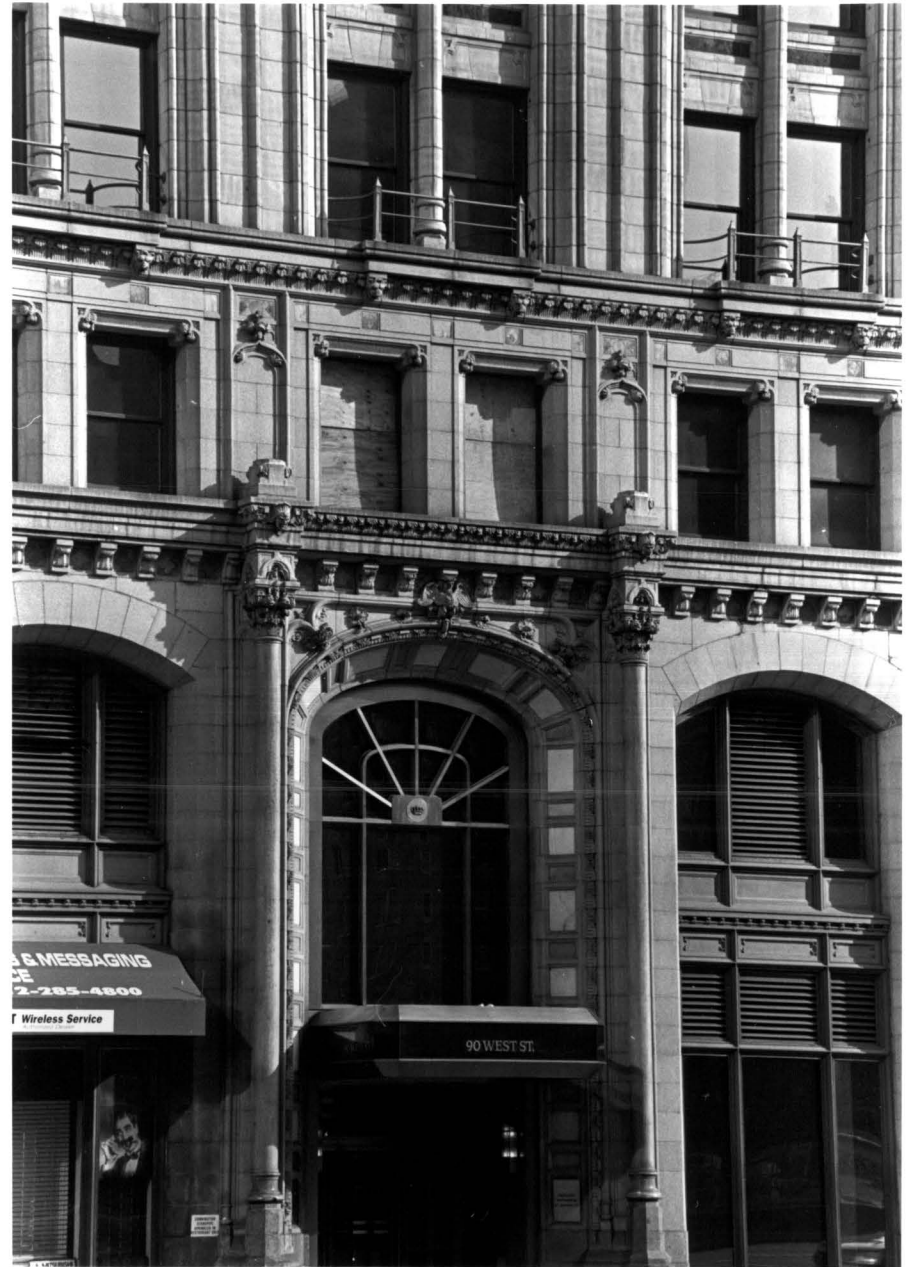
Detail of West Street entrance
