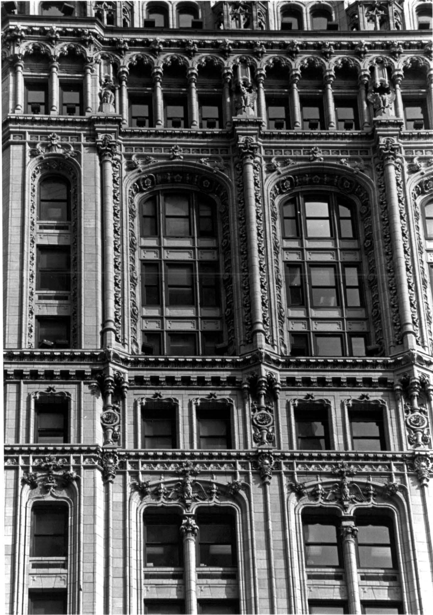
Detail of 15th through 20th floors
