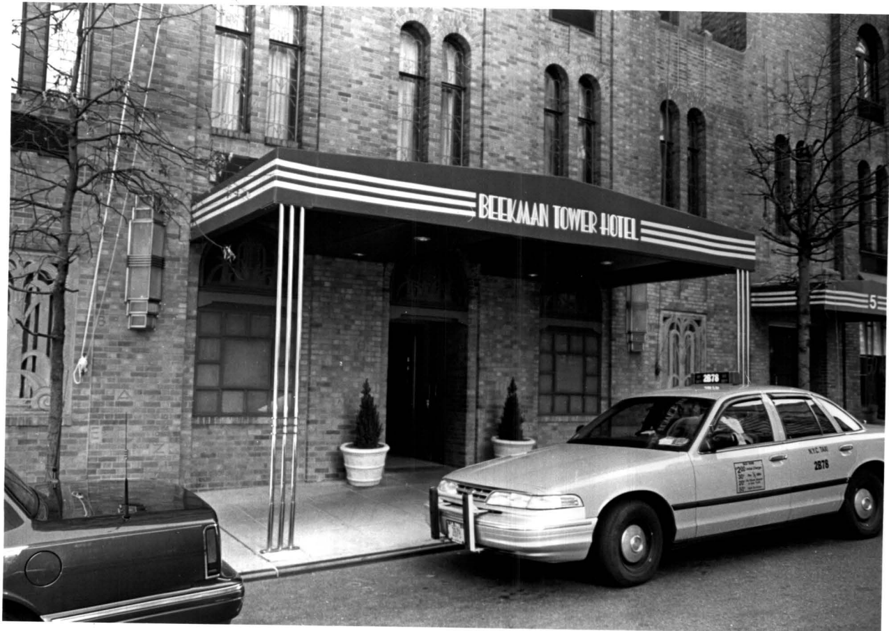
Ground story on First Avenue (top) and Mitchell Place (bottom)
